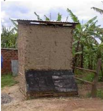
Fig. A-1: Cheap Ecosan toilet built using local materials
