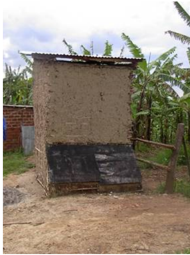
Plate 4.8: Low-cost Ecosan toilet, Costs about Ug.Shs. 80,000
