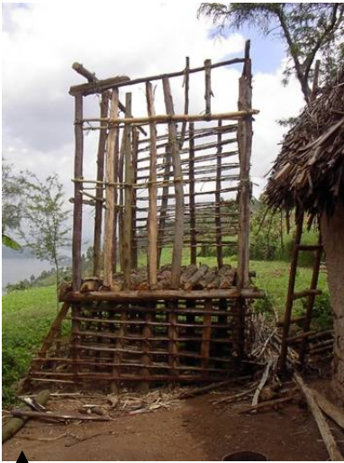
Plate 4.7: Low cost ecosan toilets. Starting it up can be built out of local materials.
