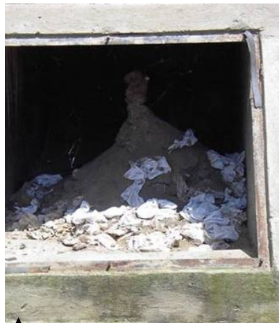
Plate 5.2: The inside of a toilet chamber. Kabale – No smell, no flies, Looks good!
