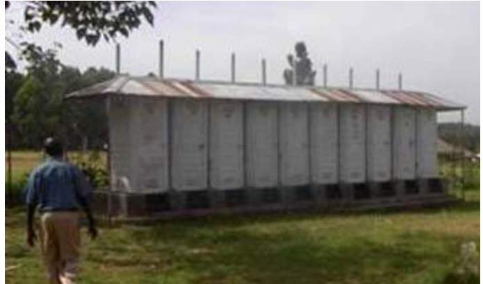
Plate 4.9: Crestank (U) factory made ecosan toilets installed at Edioffe girls secondary school, Arua
