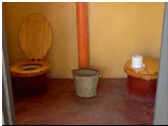
Fig. A-2: Inside an ecosan toilet that can be expensive
