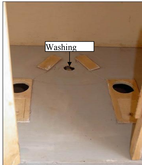
Plate 4-4: Detail of washing point
