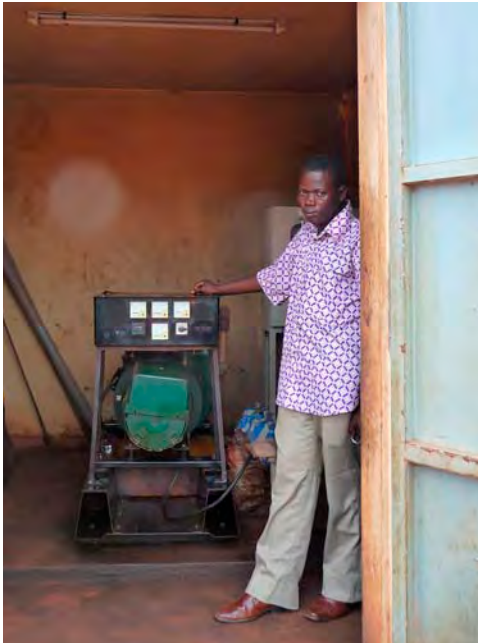
Exploitant small piped water supply system
