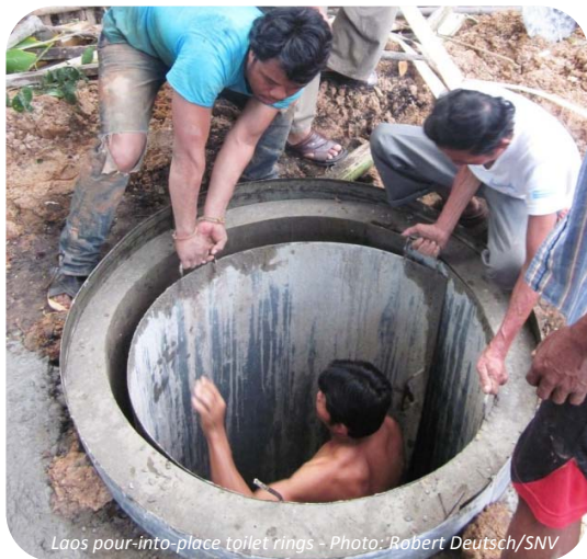
Laos pour-into-place toilet rings - Photo: Robert Deutsch/SNV
