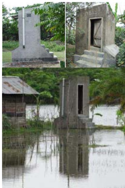
Figure 20: Design of UDDT for Flooding 18
