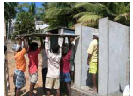
Rapid assembling of prefabricated toilet facilities made of ferro-cement
