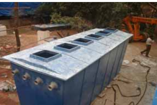
A prefabricated fiberglass DEWATS plant before installation. It is capable of serving up to 500 people.
