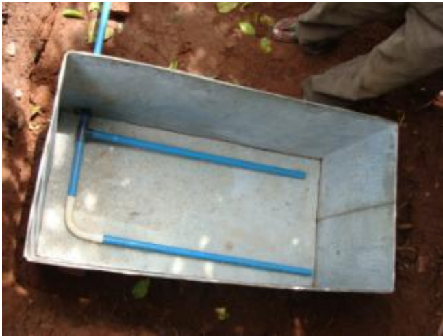
Perforated drainage pipes at base to collect filtered water. Outlet sealed with rubber washer and inner tube.
