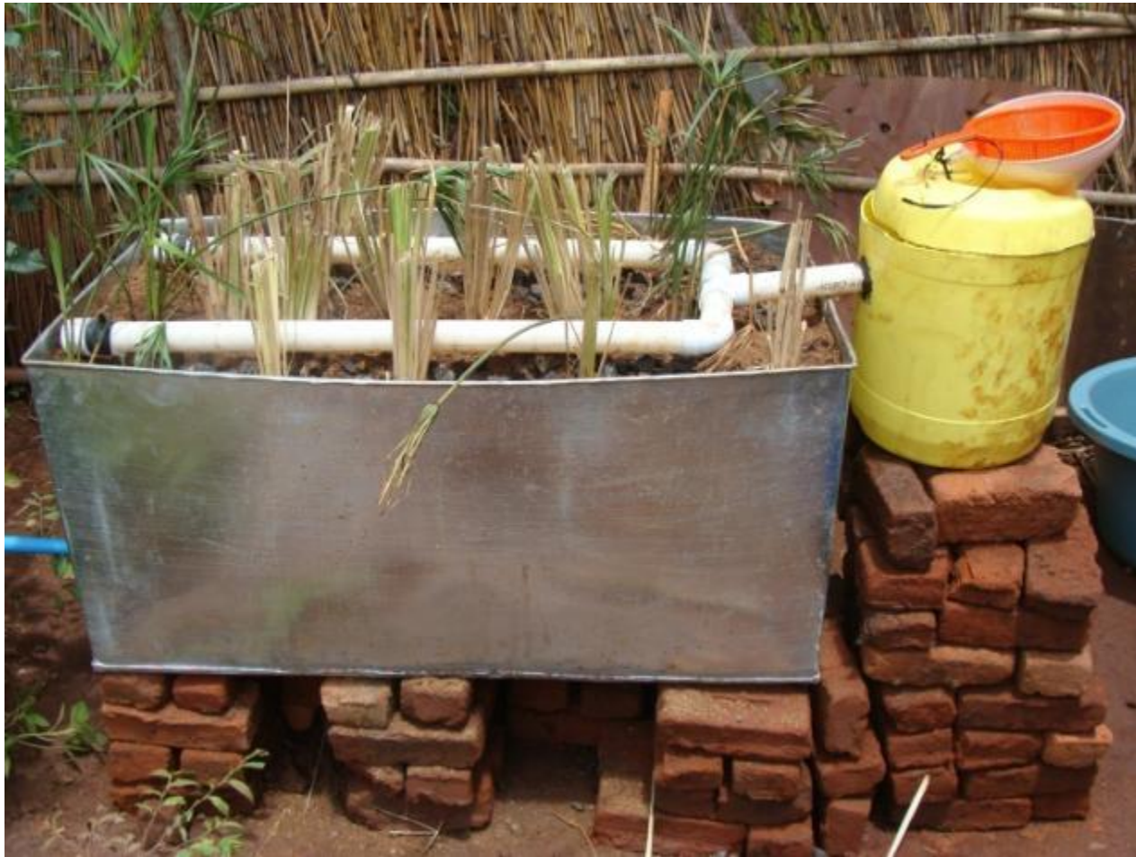
A greywater treatment system constructed in Lilongwe
