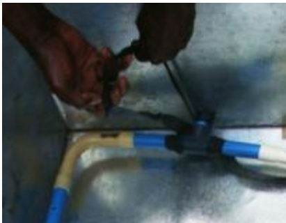
Perforated drainage pipes at base to collect filtered water. Outlet sealed with rubber washer and inner tube.
