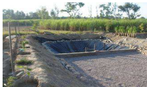
Fig. 3: The final phases of the SSF-CW
