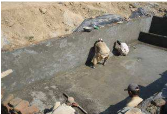
Fig 8: Construction phase of ABR showed no sign of ground water seepage
