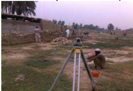
Fig. 4: Survey work for drains in progress
