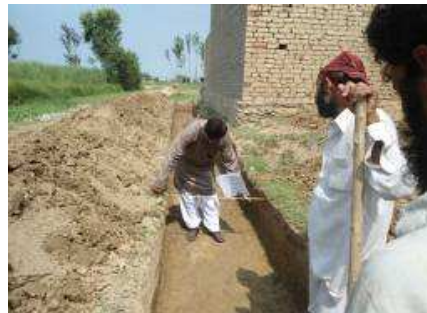
Fig. 6: Creating the drains
