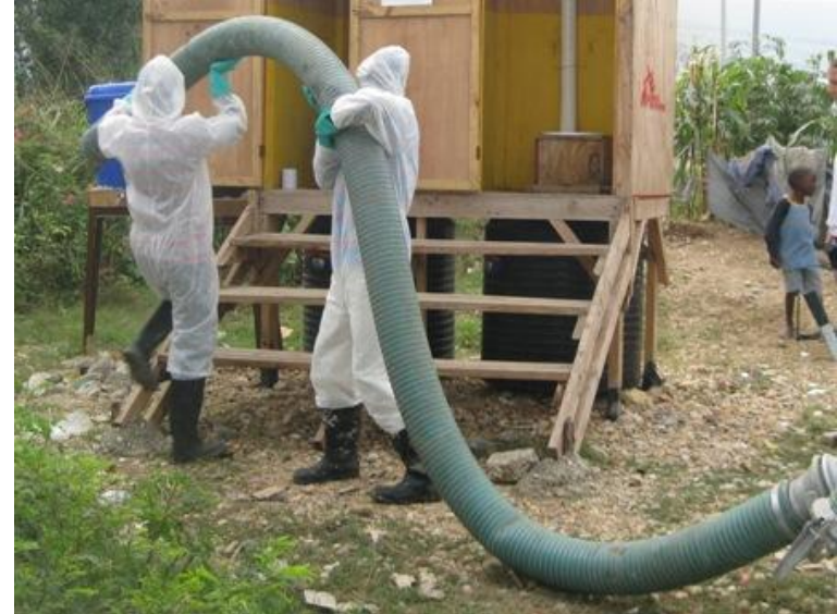
Empty pipe at end of aspiration
