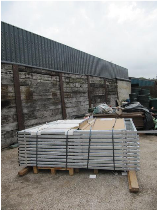
Everything needed to construct 10 cubicles minus collection vessels & plumbing
