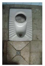
**Fig. 9:** Urine diversion squatting pans with a third outlet in the front for anal cleansing with water (source: K. Sintayehu, 2010).
