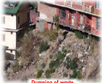
Dumbina of waste
