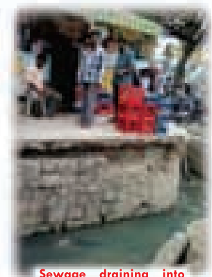
Sewage draining into storm water drains
