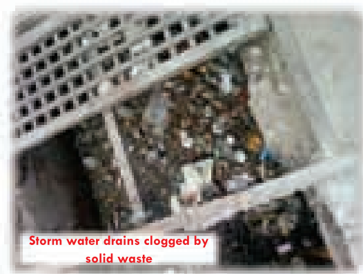
Bad condition of storm water drains
