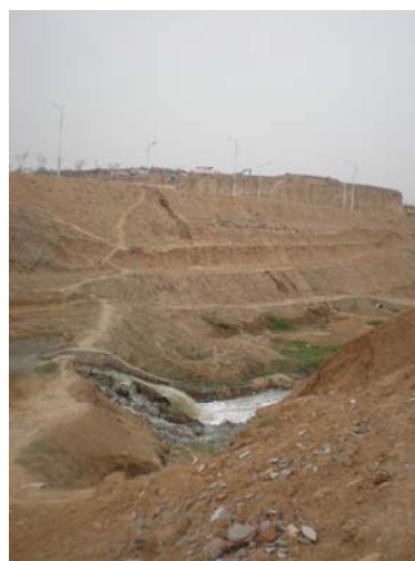
Figures 3a-b. Discharge outfalls for EETP treated greywater (left) and Dongsheng STP treated wastewater (right).
