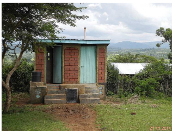
Figure 2. Double vault UDDT unit with 2 cubicles and 4 faeces vaults in Kakichuma Primary School. The hand washing tank is on the left side of the toilets, placed on the urine collection chamber. At the back of the toilet cubicle a ventilation pipe can be seen.
