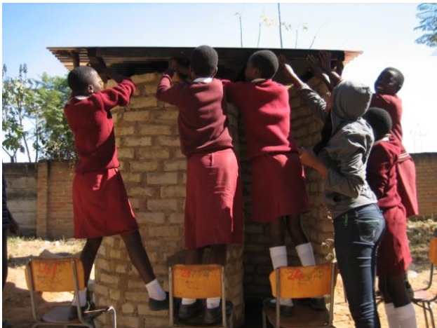
The roof must be laid square and the timbers placed on the brick wall for support.
