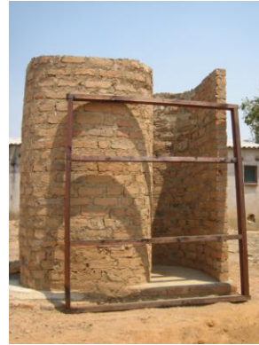
The wooden frame is nailed together and treated with wood preservative
