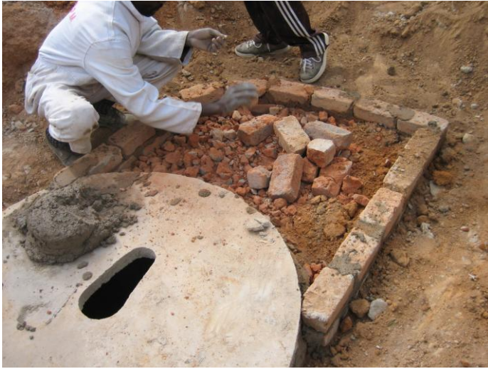
The brick are built up to slab level and the space inside filled with brick rubble and soil which is rammed hard. The slab extension is built 850mm to one side of the slab.
