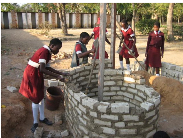
A total of 20 or 21 courses of bricks are built for the superstructure.
