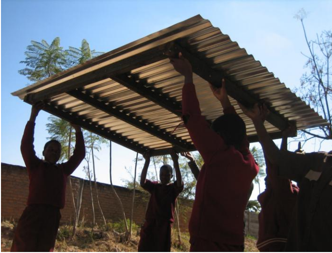
The roof lifted up and placed on the superstructure
