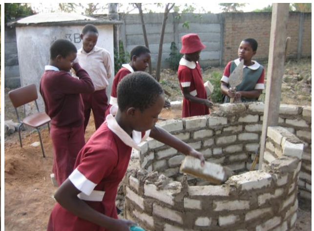
A total of 20 or 21 courses of bricks are built for the superstructure.
