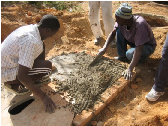
A strong mix of concrete (one part Portland cement and 5 parts river sand) is then laid over the rubble to form a floor.
