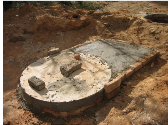
A strong mix of concrete (one part Portland cement and 5 parts river sand) is then laid over the rubble to form a floor.
