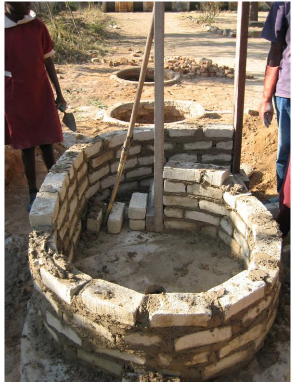
The spiral shape rising above the slab and extension.
