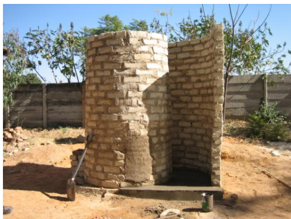
The brickwork rises and is now complete. The walls may not be perfectly upright, but the special spiral shape provided the strength. It was the first times the girls had built a toilet in this series of photos. Practice makes perfect.
