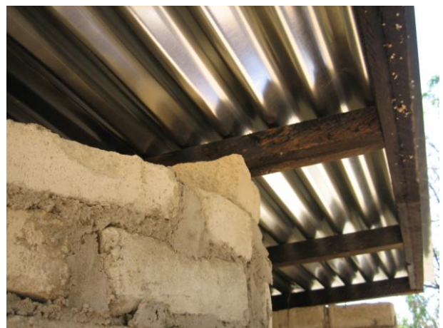
The roof must be laid square and the timbers placed on the brick wall for support.
