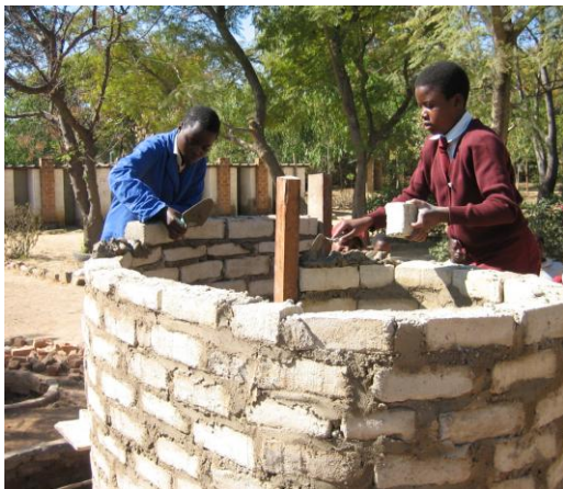
The brickwork rises and is now complete. The walls may not be perfectly upright, but the special spiral shape provided the strength. It was the first times the girls had built a toilet in this series of photos. Practice makes perfect.
