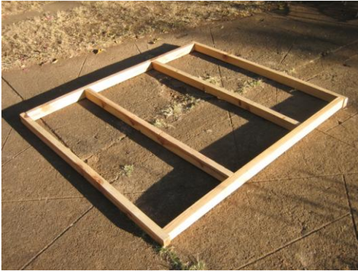
The wooden frame is nailed together and treated with wood preservative
