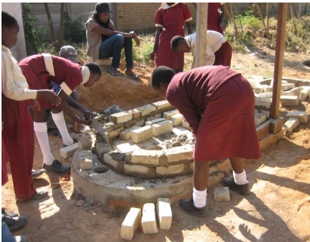
The girls can build from both ends of the spiral wall. The spiral shape gives the structure great strength even if the walls are not built perfectly straight.
