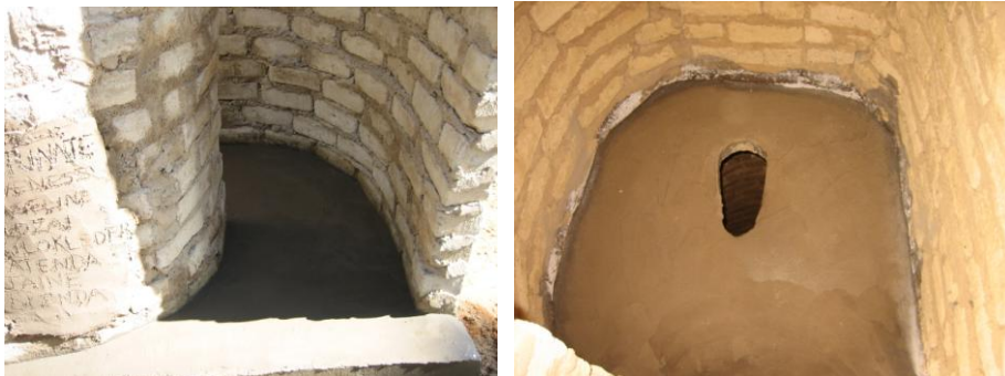
The toilet floor is laid so it slopes towards the squat hole. It is made in strong concrete and made smooth. It can be painted with a epoxy bitumen paint to reduce urine absorption.
