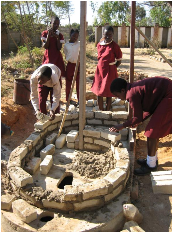
The spiral shape rising above the slab and extension.
