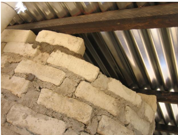
The roof must be laid square and the timbers placed on the brick wall for support.
