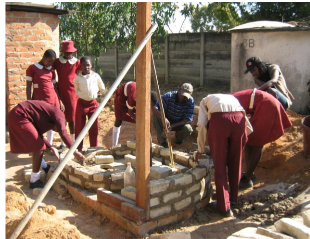
The girls can build from both ends of the spiral wall. The spiral shape gives the structure great strength even if the walls are not built perfectly straight.
