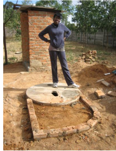
The brick are built up to slab level and the space inside filled with brick rubble and soil which is rammed hard. The slab extension is built 850mm to one side of the slab.
