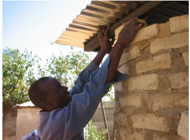
The roof must be laid square and the timbers placed on the brick wall for support.
