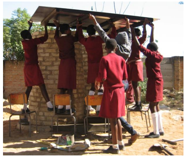
The roof lifted up and placed on the superstructure
