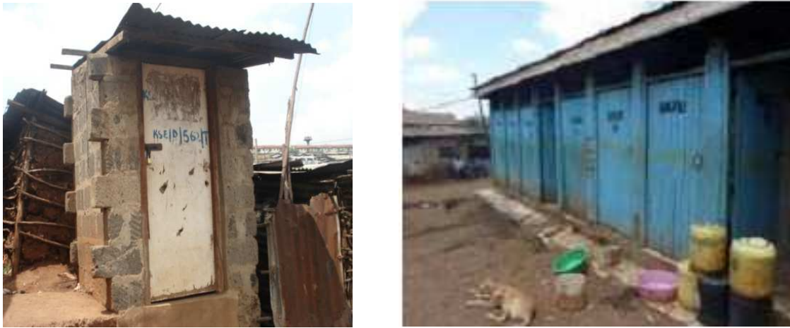
Figure 2 a – b: Shared single and community-shared multiple pit latrines
