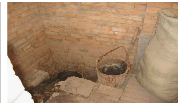
Figure 7. Buckets are used to collect excreta from all members of families which are applied to vegetable fields at periodical intervals- Xanxi province China.
