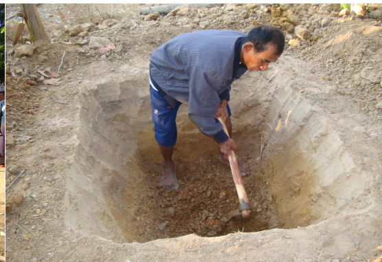
Figure 4. A man digging toilet pit immediately after CLTS triggering in a village of Cambodia.
