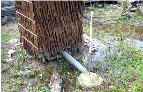
Figure 5. Toilet models developed by the ODF community in Kalimantan, Indonesia to tackle the problem of high water table and seasonal water logging. Notice how Rain-water harvesting jar is used as an underground septic tank.
