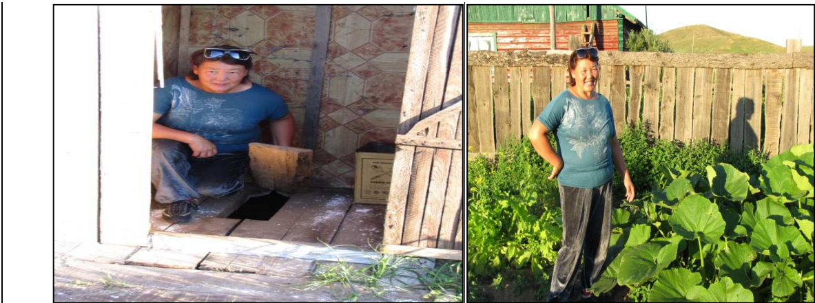
Figure 12. Dry pit latrine with retractable wooden lid cover constructed within a few days of triggering in villages in Zuunkharaa Sum in Mongolia.
