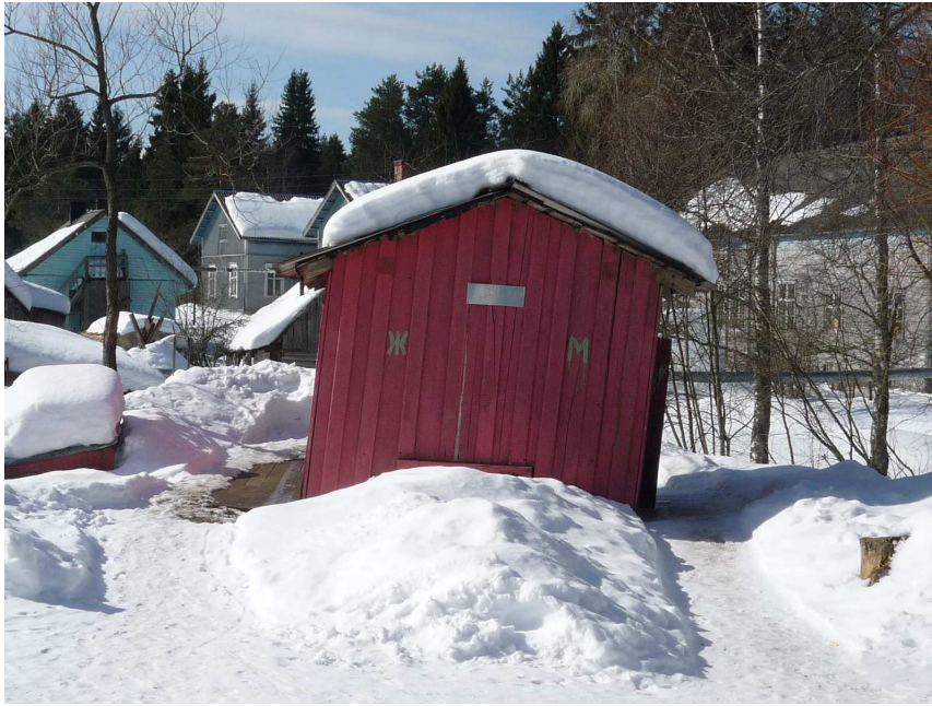
Pic. 2 The toilet construction in Harlu school
