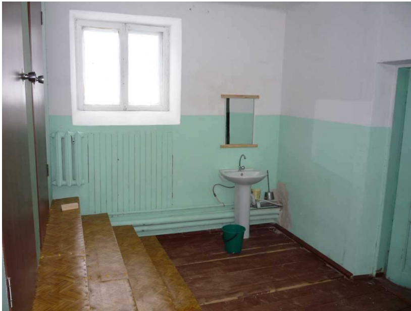
Pic. 4 The point for hand washing
