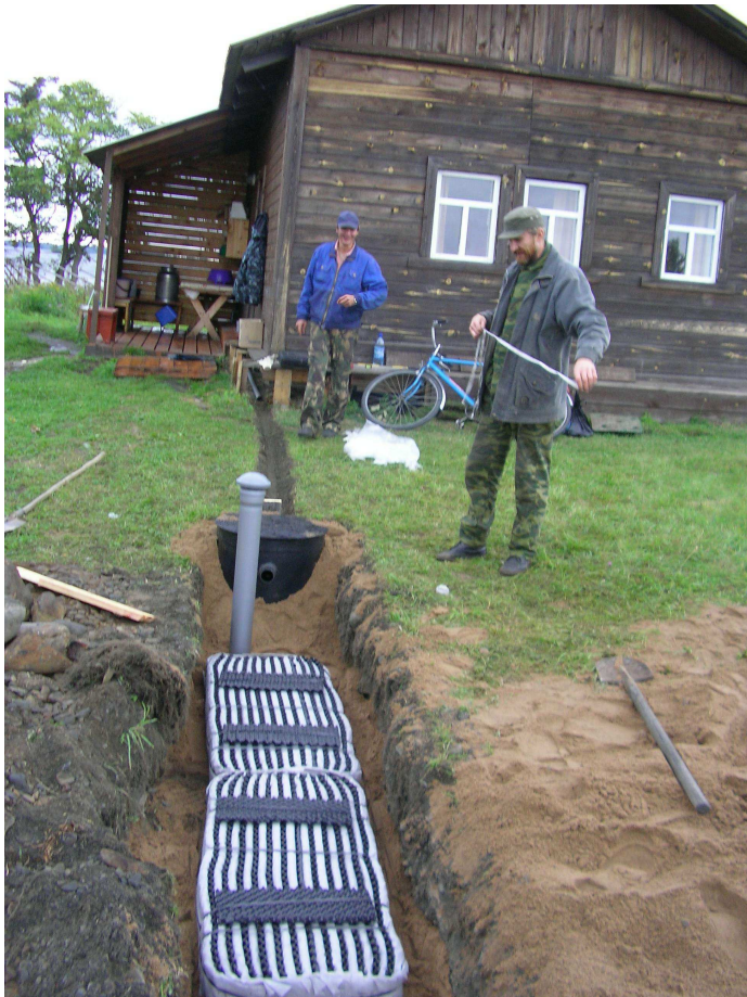
Pic. 8 The construction of the waste waters purification system
