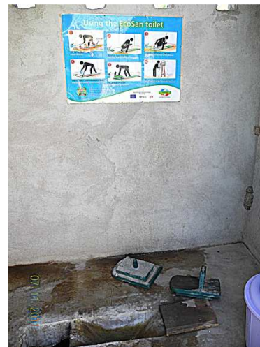
Figure 12. A view inside a UDDT cubicle, Kendu Muslim Secondary School with an explanatory poster on the wall, squatting pan with urinating hole and two holes for faeces leading to two vaults that are used alternately. On the right corner is a bucket for dehydration material, which is ash in this case.
