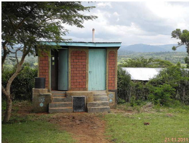
Figure 21. UDDT unit in Kakichuma Primary School. The hand washing tank is on the left side of the toilets, placed on the urine collection chamber. Behind the toilet cubicle a ventilation pipe can be seen.
