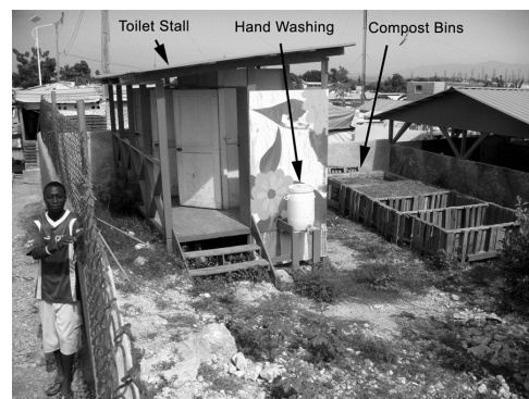
Figure 4: A toilet stall at the Amurt school, located next to the compost bins.
