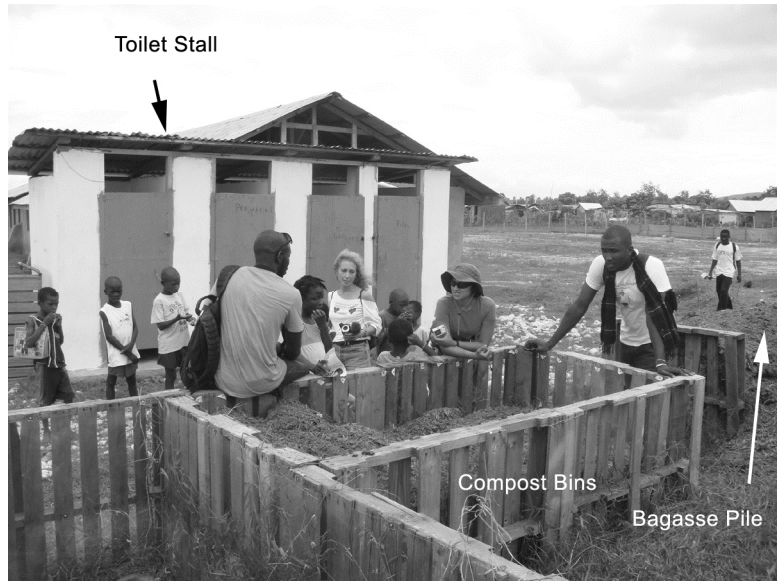
Figure 20: The toilets at the Matt Gunn orphanage site are located adjacent to the compost bins. There is no odor and no flies. A bagasse pile nearby provides the cover materials.
