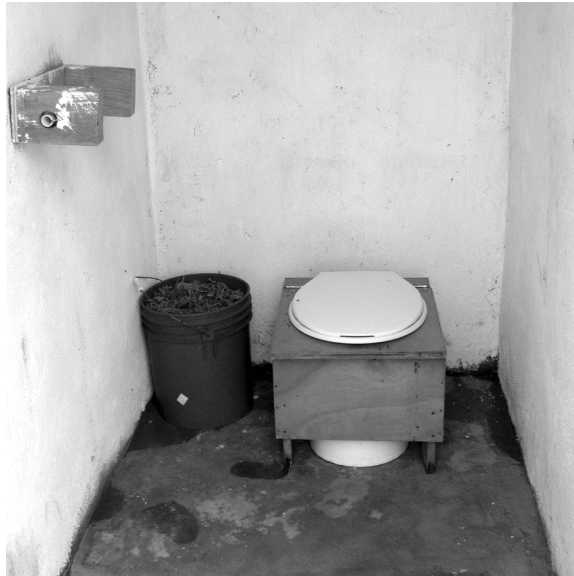
Figure 2: Toilet contents are covered inside this receptacle with sawdust and/or bagasse. The 20-liter receptacle simply lifts out when full.
