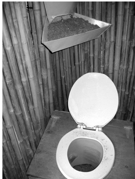
Figure 25: Sopudep uses 20 liter receptacles that lift out of the toilet when full. The bagasse is dispensed from a wall-mounted bin.
