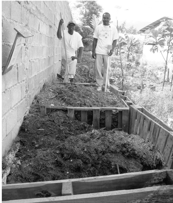
Figure 10: Two men manage the compost sanitation system at the Amurt School. The nearer bin has reached maturity and is being used in the gardens. The far bin has been aging for 6 months and is still over approximately 55C. It will require months more to reach maturity and cool down.
