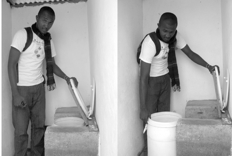
Figure 22: The Matt Gunn toilets utilize both 20 liter and 60 liter toilet receptacles. This photo shows a 60 liter toilet. The receptacle simply slides out the front of the toilet when full, and then a lid is placed on the toilet until it is emptied.
