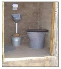
**Fig. 11**: Inside view of UDDT: urinal for men (left), bucket containing sand or ash, cover over second vault on the left side and urine diversion pedestal on the right (source: EWS).
