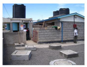
Fig. 3: New public sanitation facility with water kiosk (left side). Underground biogas plant in front.
