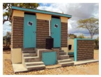
**Fig. 3** School UDDT block with two cubicles for boys with urinal on the right and hand washing station in the centre on top of the urine collection chamber at Mwala Primary School near Machakos (source: Johannes Orodi, GTZ-Kenya, Oct. 2009).
