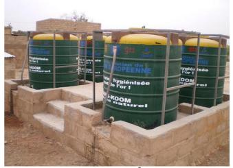
**Fig. 8:** Eco-station with four 1 m<sup>3</sup> plastic tanks for urine sanitisation (by storage over a period of one month) in sector 27 (source: A. Fall, 2009).
