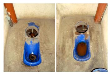
**Figure 19** Left: In the boys section piled up faeces are visible as containers are filled up, fresh faeces are not covered with ash, signs of cross-contamination in the front part. Right: Blocked urine pipe in the girls section (Source: L.Kraft, May 2011)
