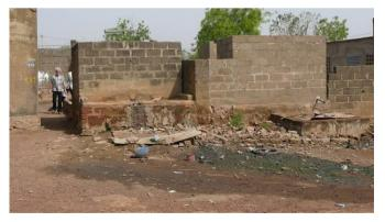
**Fig. 8:** Former desiccation (drying) chambers of UDDTs have been converted into pits to collect faeces and to be pumped empty when full (source: Stefan Hofstetter, March 2009).
