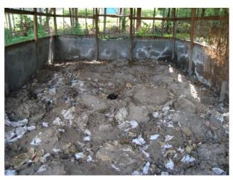
**Figure 17** Dried faeces mixed with not degradable materials inside the drying shed (Source: L.Kraft, May 2011)
