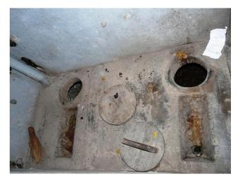
**Fig. 6**: Very dirty and not well maintained UDDT (inside), 8 years after construction. It seems that both faeces vaults are used at the same time. Note the two round wooden lids to cover the faeces holes (source: A. Leitner, 2011).
