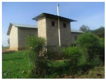
**Fig. 7**: Back view of the two UDDTs for teachers in Kiruhura primary school. At the base (covered by the bushes) are the access doors for the faeces vaults.
