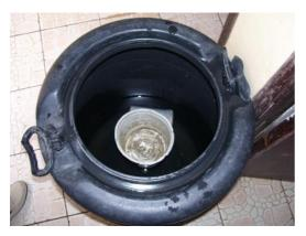
**Fig. 7:** Pour flush system with small bucket (2-4 L) in drum. The small bucket is used to flush the toilet.
