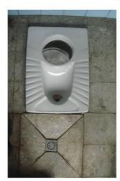
**Fig. 7:** Urine diversion squatting pans which an extra outlet in front for anal cleansing with water. (source: K. Sintayehu (2010)).
