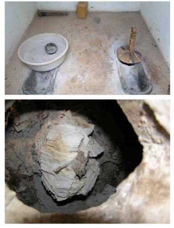
**Fig. 6:** (Top) Doubled chambered UDDT with only one chamber in use at a time. The other source separation pan is kept covered. (Bottom) Ash and toilet paper used for drying material. (Source: Hans Schattauer, 2012)
