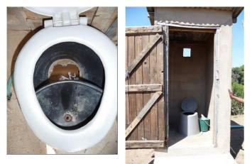
**Fig. 7:** Left: UDD toilet working properly in West Hanahai. Right: This UDDT was well maintained, ash standing next to the toilet and composting unit filled (in Paje).
