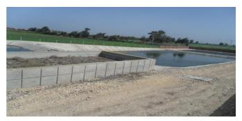
**Fig. 8:** Treatment plant of Moufty El-Kobra, with the three stabilisation ponds. In the forefront, the sludge drying bed is seen (source: N. Stuber; 2010).
