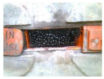
**Fig. 14** A urine pipe of a urine diversion squatting pans got blocked with ash at Muslim Primary School, Mumias. Faeces drop holes are covered with lids on the left and right in this photo (source: Laura Kraft, GTZ, June 2010).
