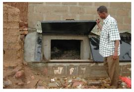
**Fig. 5:** Faeces vault of UDDT with opening to remove the dried faeces (source: GTZ, 2002).
