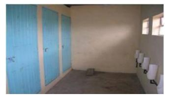
**Figure 8** Inside the boys' toilet - 3 cubicles (left) and 6 waterless urinals (right) made of plastic buckets (Source: Muchiri, 2009)
