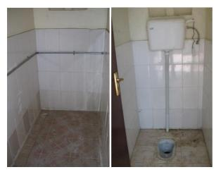
**Fig. 6:** Left: Urinal using a tiled wall (no door) with optional water flush. Right: Squatting pan with 10 L cistern (flush toilet); but these days a manual pour flush system is used for toilet flushing (see Fig.7).
