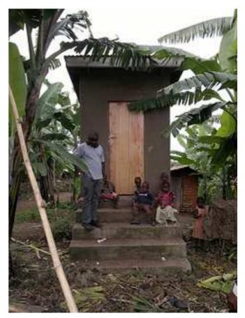
**Fig. 5:** UDDT constructed for a household where the by products from the toilet are reused in the surrounding banana plantation. The UDDT was built a part of the Ecosan program. (Source: Hans Schattauer, 2012)
