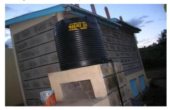
Fig. 8 Roof water harvesting system for hand washing at the new UDDT.
