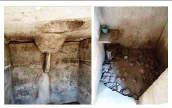
**Fig. 9**: Situation 8 years after construction: Left: walls of faeces vault with deep cracks. Right: bathing cubicle's concrete floor is broken (source: A. Leitner, 2011).
