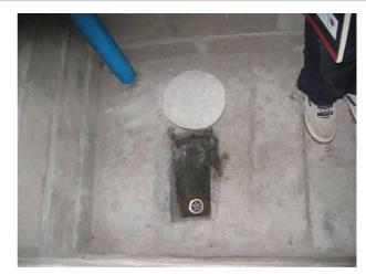
**Fig. 5:** Inside a *new* UDDT; the faeces hole is covered with a lid; the urine separation part is fitted with a sieve. You can see the ventilation pipe at the back left (source: M. Fogde, 2003).
