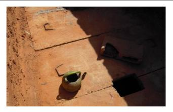
**Fig. 8:** The slabs of the pit latrines, drop hole is at the bottom right in the shaded part of the photo (source: Mahamat Absakine (2010) Groupe URD). When the document is printed black and white, the drop hole is not visible. Use better photo?
