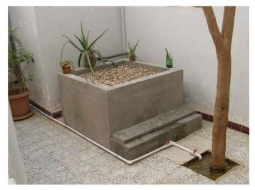
**Fig. 10:** The rebuilt greywater filter at the project offices in Béni Abbès (source: AHT GROUP AG, 2011).
