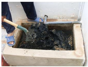
**Fig. 9:** Excavation of the completely clogged filter media in the original (source: AHT GROUP AG, 2011).
