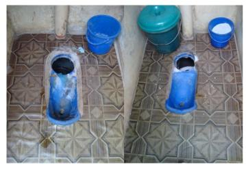
**Fig. 14** On the left, inside view of toilet used by men with empty ash container, urine on the floor and signs of faecal cross-contamination. Right: Inside view of toilet used by women (Source: L. Kraft, May 2011)
