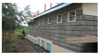
Figure 11 Ventilation pipes and windows for each UDDT collection vault and cubicle respectively (Source: Muchiri, 2009)
