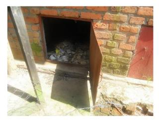
**Fig. 10:** Open vault of a UDDT in Kiziguro primary school. Paper is used as cleansing material.
