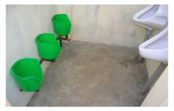
**Fig. 7** Inside the men's urinal showing the fabricated plastic containers urinal for the kids and standard ceramic urinals.
