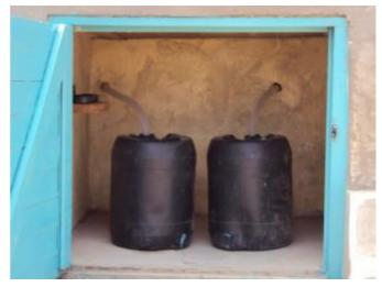
**Fig. 11** Two 20 L urine containers with flexible hoses in a vault attached to the UDDT at Mwala Primary School, Ukambani (source: Johannes Orodi, GTZ Kenya, Oct. 2009).
