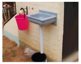
**Fig. 6:** Basic handwashing facilities attached to the toilets. The pink bucket provides fresh water, the cup is used to fill the basin and the black bucket collects the greywater which can be used for irrigation (source: GIZ, Kleemann, 2011).
