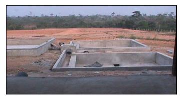
Fig. 4: Faecal sludge drying beds (source: Olufunke Cofie, 2002).
