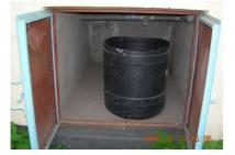
**Figure 10** Interior of a faeces collection vault with a 50 litre container to collect the faeces (Source: Muchiri, 2009)
