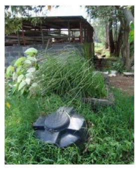
Figure 18 Greywater treatment system with settlement tank (Source: L.Kraft, May 2011)
