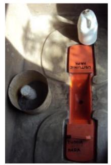
**Fig. 7** Plastic urine diversion squatting pan with concrete footsteps inside a UDDT. Urine is collected in the centre; the two lids are covering the two faeces vaults (source: Laura Kraft, GTZ, June 2010).
