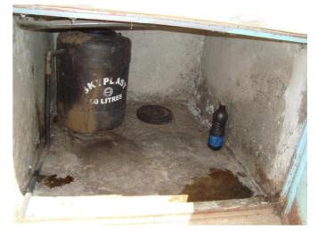
Fig. 12 50 liter urine tank with small leakage in pipe (L.Kraft, May 2011)
