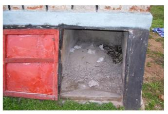
**Fig. 7:** Faeces collection vault which is half full (source: David Watako, GTZ-Kenya, July 2009). Note: Sufficient use of ash and appropriate use results in a dry and odour free condition of the vault.
