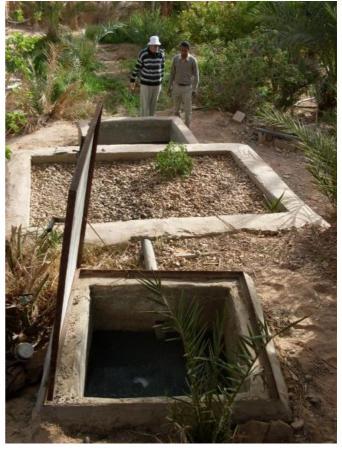
**Fig. 8:** The grease trap /settlement basin, filter and storage tank for the irrigation of the vegetable garden and the house of Mr. Boussouri (garden visible in the background) (source: AHT GROUP AG, 2011).
