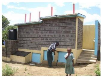
**Fig. 11** The rear of the UDDT showing the single vaults and the solar drier for the double vault
