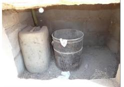
**Fig. 6:** Collection chamber under a properly working ecosan UDD toilet (left: urine container, right: faeces bucket) in Paje.
