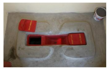
**Fig. 8:** Inside view of a UDDT with ash container on the right. The squatting pan has two faeces outlets: only the one on the left is currently in use. In the left corner is the ventilation pipe (not visible) (source: Moses Wakala, GTZ-Kenya, June 2008).
