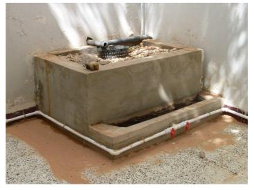
**Fig. 4:** The first pilot greywater filter and reuse system installed at the project offices (source: AHT GROUP AG, 2011).
