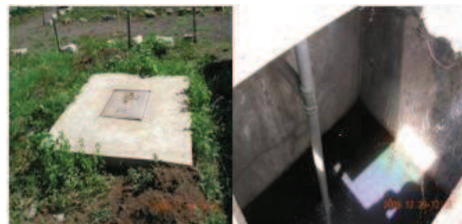
Figure 12 Urine collection tank (2000 L) at Crater View secondary school (Source: Muchiri, 2009)
