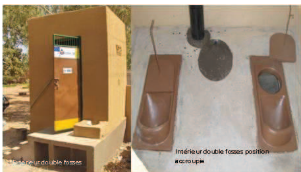
Fig. 7: Outside and inside views of a double vault UDDT with urine diversion squatting pans and anal wash area (dark circle in the middle). Urine jerrycans are stored under the stairs (left picture) (source: CREPA, 2008).
