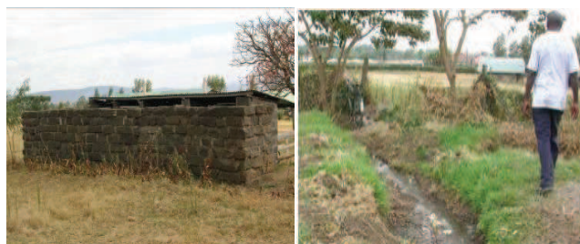
Figure 4 Left: The old pit latrines at Crater view secondary school (Source: Muchiri, 2008) Right: Greywater from kitchen and dish washing was disposed in open drains prior to the project (Source: Raude, 2009)
