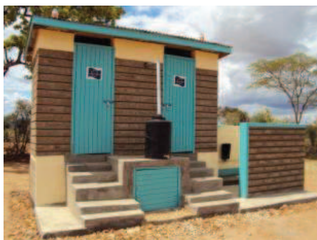
Fig. 3 School UDDT block with two cubicles for boys with urinal on the right and hand washing station in the centre on top of the urine collection chamber at Mwala Primary School near Machakos (source: Johannes Orod, GTZ-Kenya, Oct. 2009).
