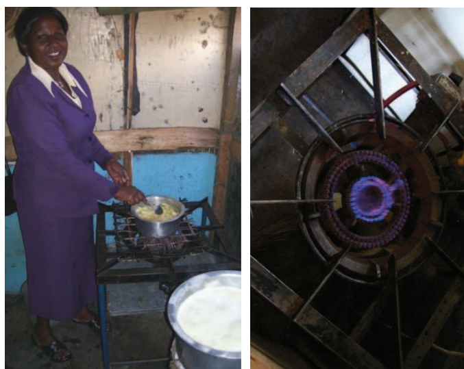
Fig. 12: Biogas is used to cook snacks and tea at the adjacent cafe.
