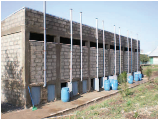
Fig. 6: Back view of the UDDT block showing vent pipes and doors to faeces vaults, Ethiopia. (source: K. Sintayehu (2010))
