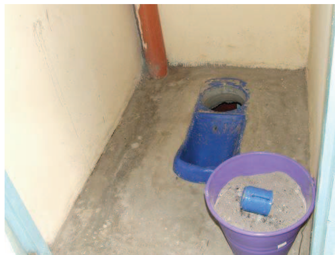
Figure 7 Inside of the UDDT, showing urine diversion squatting pan and bucket of ash (Source: Muchiri, 2009)
