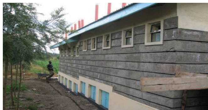
Figure 11 Ventilation pipes and windows for each UDDT collection vault and cubicle respectively (Source: Muchiri, 2009)
