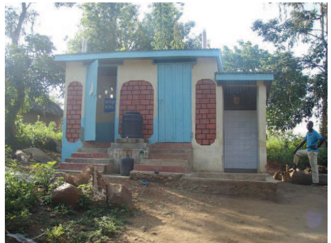
Fig. 16: A double door UDDT with attached shower for a family with more than 20 users in Western Province. The shower was added on initiative of the toilet owner (source: Laura Kraft, 2009)
