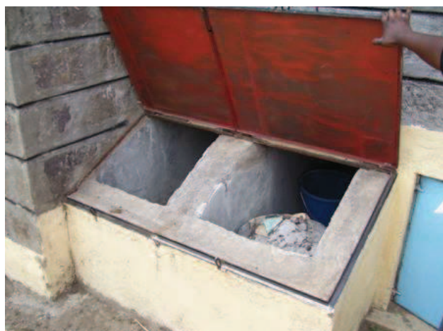
Fig. 13 Containers are placed in the solar drier of the double vault compartment (Source: Steffen Blume, 2009)
