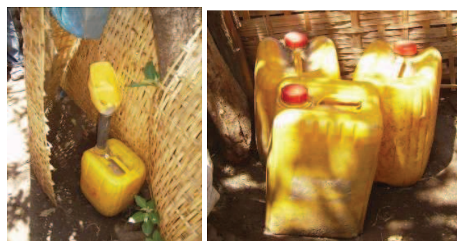
Fig. 9: Waterless urinal (source: ROSA project Arba Minch, 2009).
