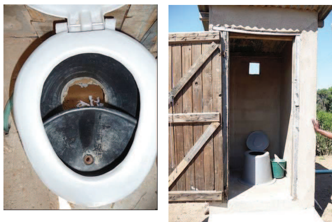
Fig. 7: Left: UDD toilet working properly in West Hanahai. Right: This UDDT was well maintained, ash standing next to the toilet and composting unit filled (in Paje).
