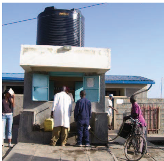
Fig. 5: Customers of the water kiosk. The water tank on the roof holds 5 m 3 (or 250 jerry cans) to bridge water supply gaps for a period of about 1-2 days.
