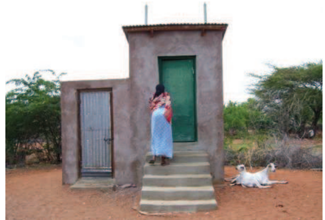
Fig. 5: Household UDDT and shower on the left in the semi-desert area of Wajir, North Eastern Province (source: Paul Mboya, GTZ-Kenya, March 2009).
