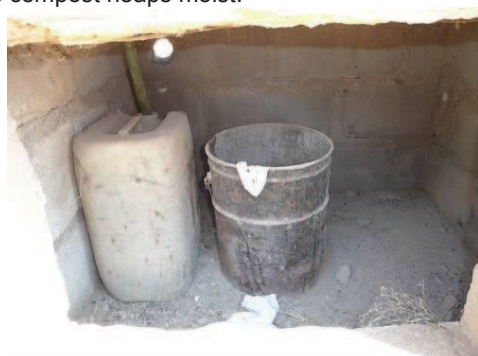
Fig. 6: Collection chamber under a properly working ecosan UDDT toilet (left: urine container, right: faeces bucket) in Paje.
