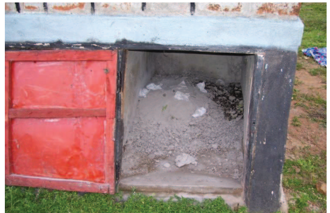
Fig. 7: Faeces collection vault which is half full (source: David Watako, GTZ-Kenya, July 2009). Note: Sufficient use of ash and appropriate use results in a dry and odour free condition of the vault.
