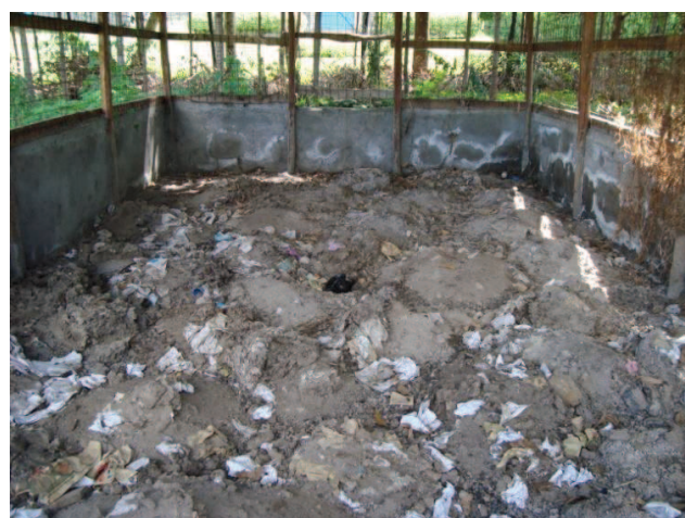
Figure 17 Dried faeces mixed with not degradable materials inside the drying shed (Source: L.Kraft, May 2011)
