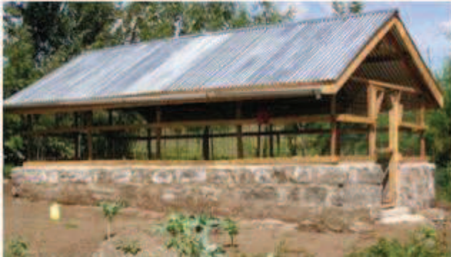
Figure 13 Drying shed for processing faecal matter from the UDD toilets (area 6 m x 3.6 m) (Source: Muchiri, 2009)
