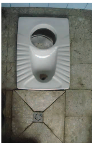
Fig. 7: Urine diversion squatting pans which an extra outlet in front for anal cleansing with water. (source: K. Sintayehu (2010)).
