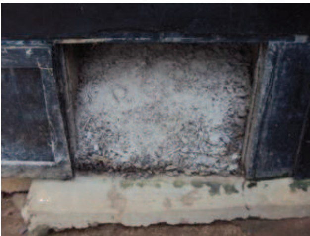
Fig. 8 Faeces vault of UDDT with ash-covered dried faeces (source: Laura Kraft, GTZ, June 2010).
