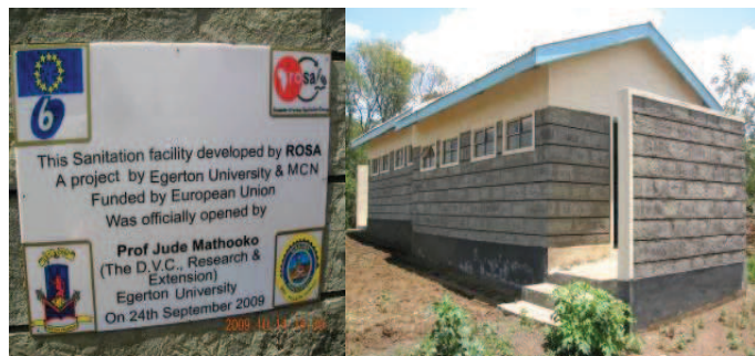
Figure 5 New school toilet implemented by ROSA project (Source: Muchiri, 2009)
