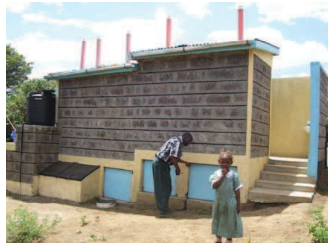
Fig. 11 The rear of the UDDT showing the single vaults and the solar drier for the double vault
