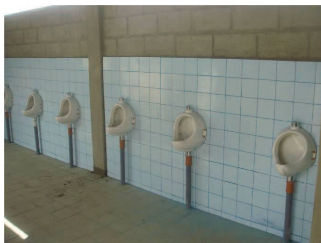
Fig. 8: The urinals of the UDDT facility at AU (source: K. M. Sintayehu, 2010).
