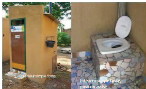
Fig. 3: Outside and inside views of a single vault UDDT constructed at town halls in Ouagadougou (with urine diversion seat) (source: CREPA, 2008).
