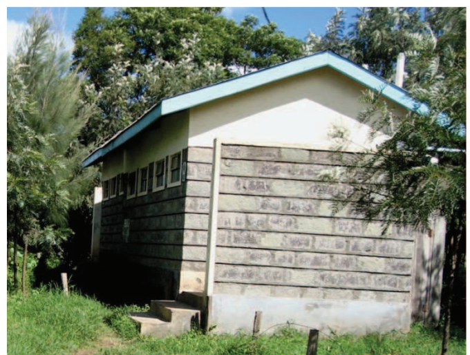
Figure 3 The UDDT facility at Crater View Secondary School two years after construction (Source: L.Kraft, May 2011)
