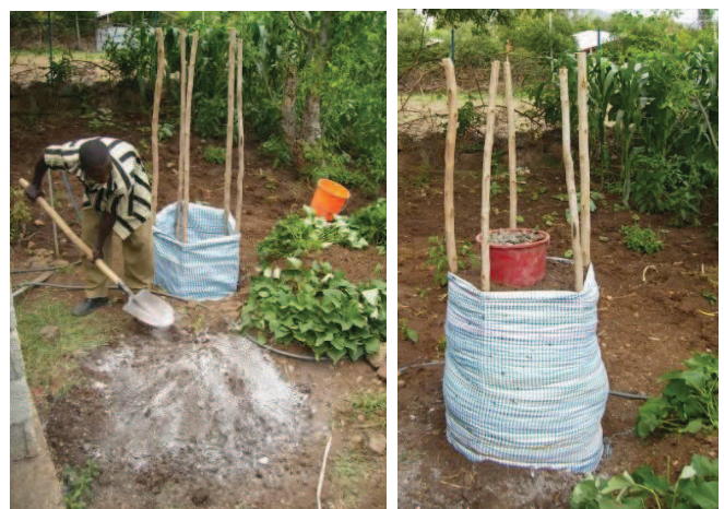
Fig. 6: Left: Mixing soil, compost and ash to fill the tower. Right: Filled greywater tower.
