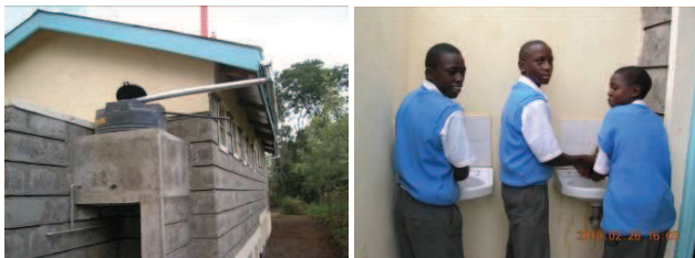
Figure 14 Roof water harvesting system and students washing their hands after visiting toilet (Source: Muchiri, 2009)
