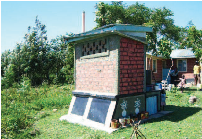
Fig. 6: Back view of household UDDT near Bungoma town in Western Province with two faeces vaults and ventilation pipe (source: Moses Wakala, GTZ-Kenya, Jan. 2010). Note: The inclination of faeces vault doors is not necessary for proper function – see Section 11. Moreover note the toilet is in relative close distance to house.
