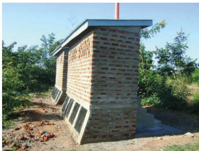
Fig. 10 Rear view of 2 toilet blocks with inclined vault doors and ventilation opening which also provide additional light inside the cubicle (source: Paul Mboya, GTZ Kenya, Jan 2009)
