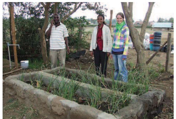
Figure 16 Greywater treatment system at Crater View Secondary School (Source: Laura Kraft, 2009)
