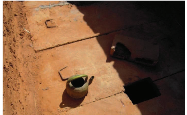
Fig. 8: The slabs of the pit latrines, drop hole is at the bottom right in the shaded part of the photo (source: Mahamat Absakine (2010) Groupe URD). When the document is printed black and white, the drop hole is not visible. Use better photo?
