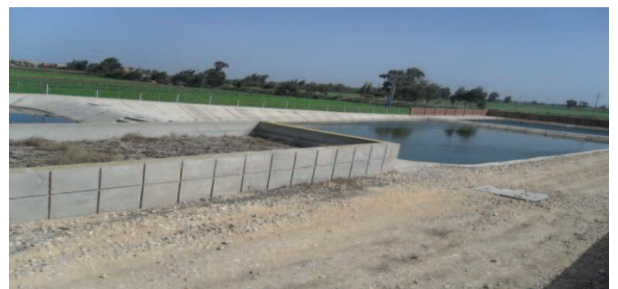
Fig. 8: Treatment plant of Moufty El-Kobra, with the three stabilisation ponds. In the forefront, the sludge drying bed is seen (source: N. Stuber; 2010).
