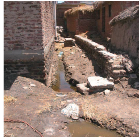
Fig. 5: Wastewater in the streets of El-Moufty El-Kobra before the project in 2002, a common situation in the villages of the Nile Delta (source: GIZ; 2002).
