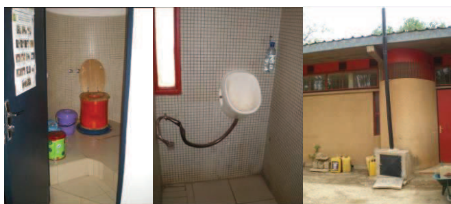
Fig. 6: UDDT inside a house (inside, backside view and waterless) (source: A. Fall, 2010).
