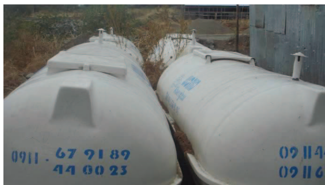
Fig. 9: Long-term urine storage tanks for UDDT at AU, Ethiopia. (source: S. Kore (2012)).
