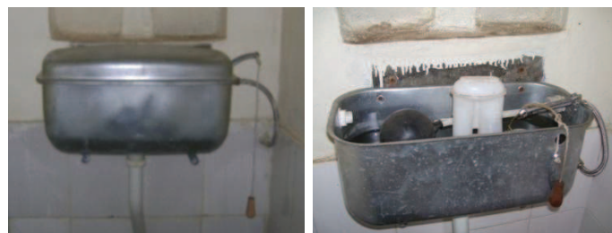
Fig. 13: Cistern after installation (left) and after vandalism/misuse and theft (right) a few weeks later. Repairs were undertaken by WSP, but the toilet operator now shifted to a pour flush system.
