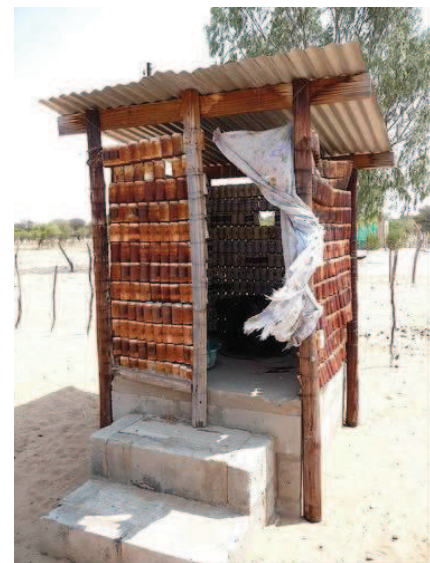
Fig. 5: Ecosan UDD toilet built out of beer cans in Hanahai. The most creative superstructure in the region!
