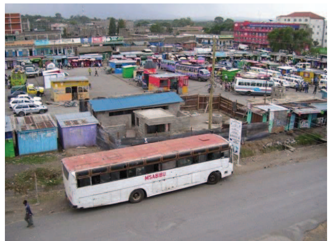
Fig. 3: View of Naivasha bus park with the public toilet at the front of the plot (behind the large bus); during the construction in mid 2007. All photos in this document by C. Rieck (GTZ) in 2008/2009.
