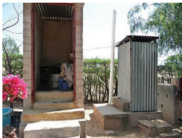
Fig. 9: UDDT (on the left) next to a pit latrine on the right (in Paje). The UDDT was never used since its installation in 2004 (as the main female of the household objects to having to empty the faeces container. The pre-existing pit latrine is used instead (when it is full, a new pit will be dug).
