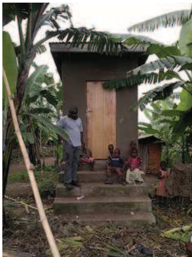
Fig. 5: UDDT constructed for a household where the by products from the toilet are reused in the surrounding banana plantation. The UDDT was built a part of the Ecosan program. (Source: Hans Schattauer, 2012)
