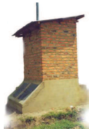
Fig. 3: An ecosan toilet (UDDT) in a household (source: Project Album, 2005).
