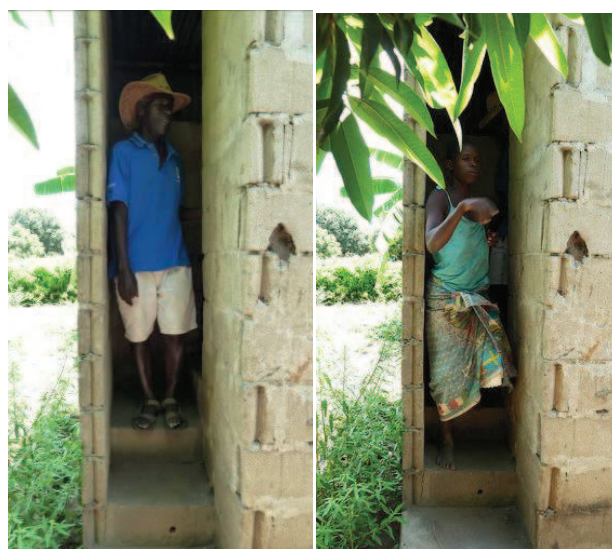
Fig. 10: The entrance to the UDDTs is very narrow (source A. Leitner, 2011).
