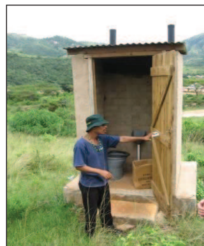
Fig. 5: Double vault UDDT in Maphephetheni in the eThekweni rural area (source: EWS).
