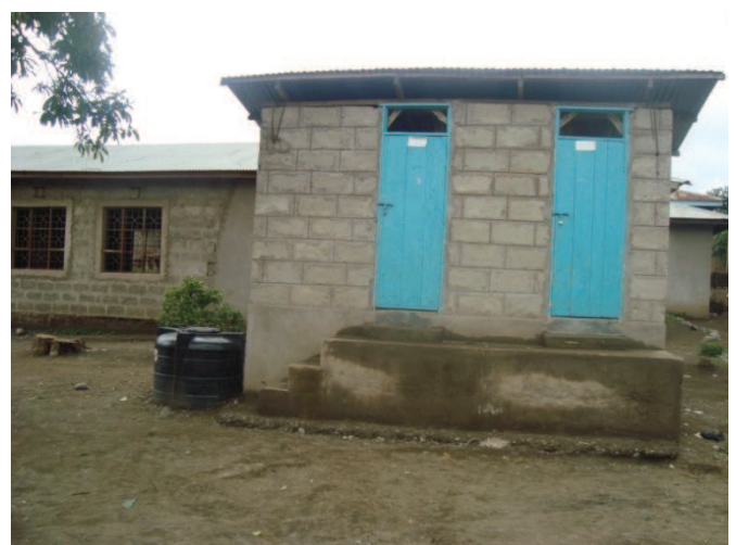
Fig. 3: UDDT toilet block (2 cubicles with 2 vaults each) made of concrete blocks in Daraja II primary school. The plastic tank for urine collection can be seen on the left side of the toilet. All pictures in this document are from the ROSA project in Arusha 2008-2010.
