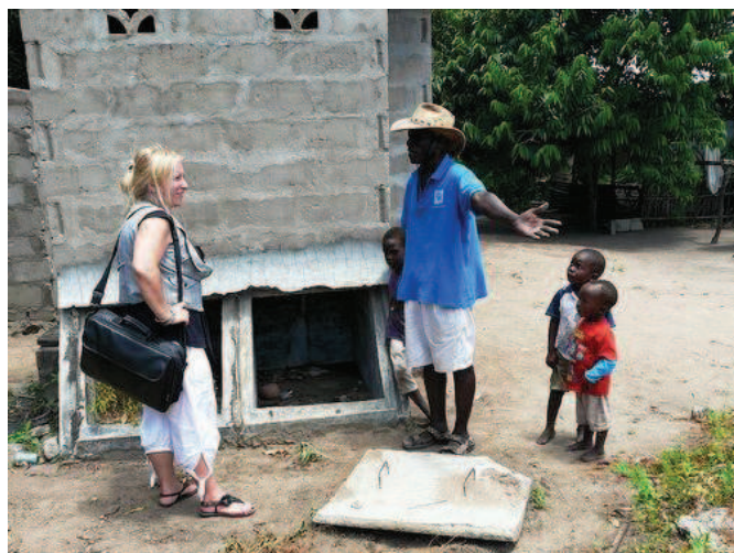
Fig. 11: Discussions about the current state of the UDDTs. This UDDT is no longer in use, note empty faeces vaults and the vault cover on the ground (source: A. Leitner, 2011).
