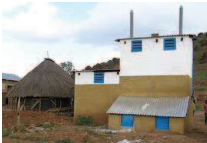
Fig. 4: Household UDDT constructed next to traditional house in semi-urban areas (Source: Hans Schattauer, 2012)
