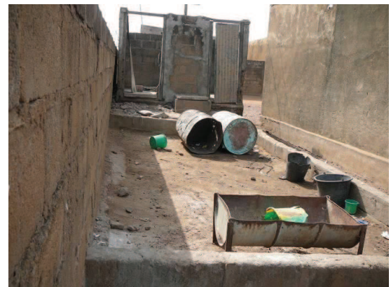
Fig. 7: A former greywater garden, which was once planted with lots of banana plants (source: Stefan Hofstetter, March 2009).
