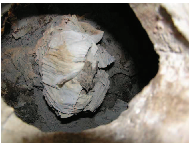
Fig. 6: (Top) Doubled chambered UDDT with only one chamber in use at a time. The other source separation pan is kept covered. (Bottom) Ash and toilet paper used for drying material. (Source: Hans Schattauer, 2012)
