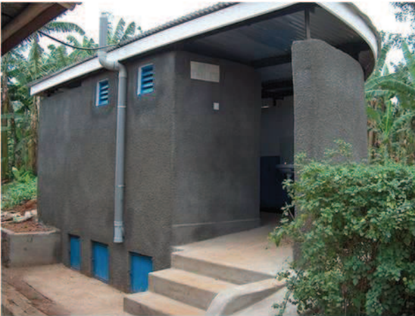
Fig. 6: Demonstration UDD toilet for teachers and visitors, five years old (source: EcoSan Club, 2009).
