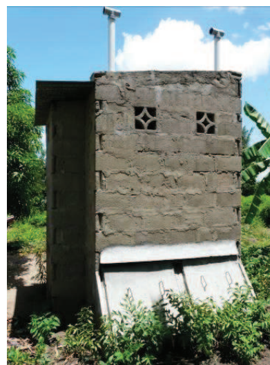
Fig. 12: Household UDDT in good condition, 8 years after construction; note metal faeces vault covers are still in place (source: A. Leitner, 2011).
