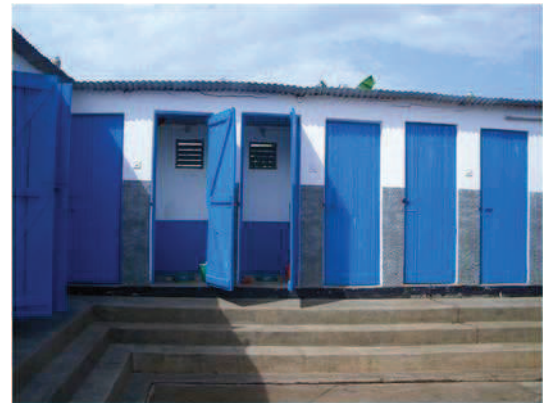
Fig. 4: New students' toilets (45 UDDTs) - these are now five years old and still in perfect condition (source: EcoSan Club, 2009).
