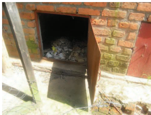
Fig. 10: Open vault of a UDDT in Kiziguro primary school. Paper is used as cleansing material.
