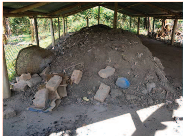
Fig. 13: Covered drying area for collected dried faeces from UDD toilets (source: EcoSan Club, 2009).
