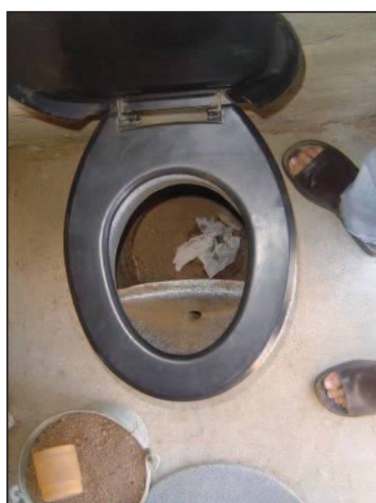
Fig. 12: Interior of a UDDT with sand container on the bottom left and plastic urine diversion pedestal from Atlas company at the top (source: EWS).
