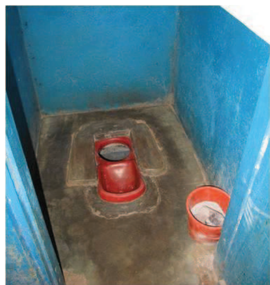
Fig. 5: Interior of a UDD toilet for students, showing UD squatting pan after approx. five years of use (source: EcoSan Club, 2009).
