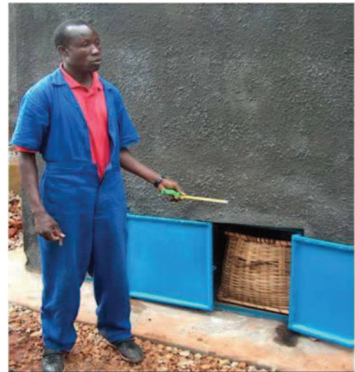
Fig. 8: Wooden faeces collection basket in vault of UDDT. In front Alex Oryem, the site engineer from Norman Construction (source: EcoSan Club, 2005).
