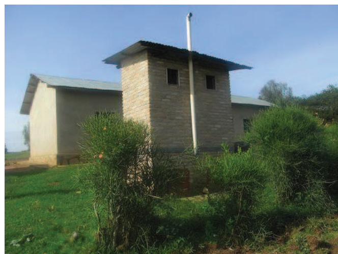
Fig. 7: Back view of the two UDDTs for teachers in Kiruhura primary school. At the base (covered by the bushes) are the access doors for the faeces vaults.
