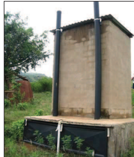
Fig. 7: Back view of double vault UDDT showing access doors to two vaults and ventilation pipes (source: EWS).
