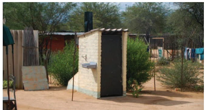
Fig. 3: Otji toilet with attached hand washing basin (source: GIZ, Kleemann, 2011)
