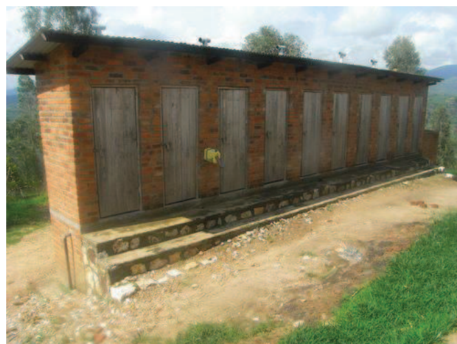
Fig. 6: Toilet block with 10 UDDTs built in Kiziguro primary school (teachers have another 2 UDDTs built separately). Five cubicles are for boys, five for girls.
