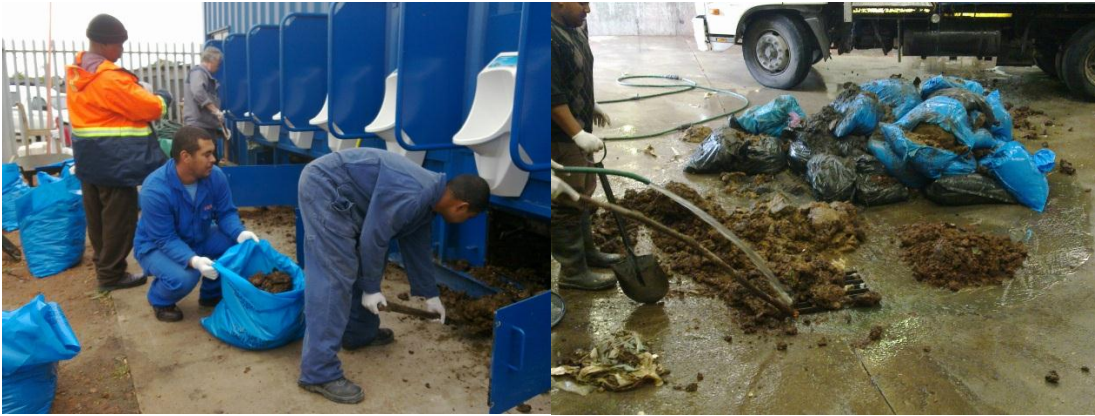
Figure 4: Bagging of faecal sludge
