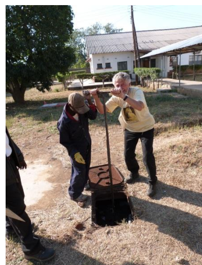
Figure 3.1 – Inspection of ST5 with metal pole. © Mirco Keller.
