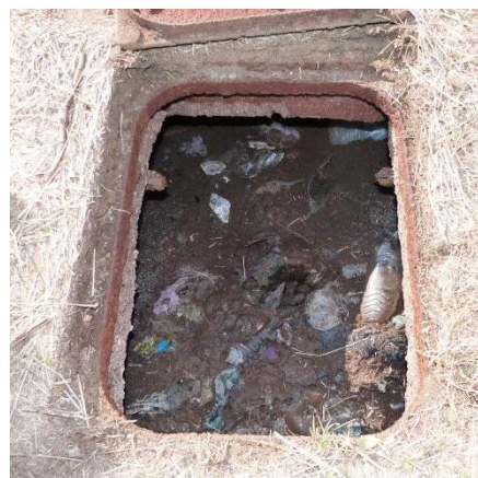
Figure 5.3 – Solidified sludge of ST5. © Mirco Keller.
