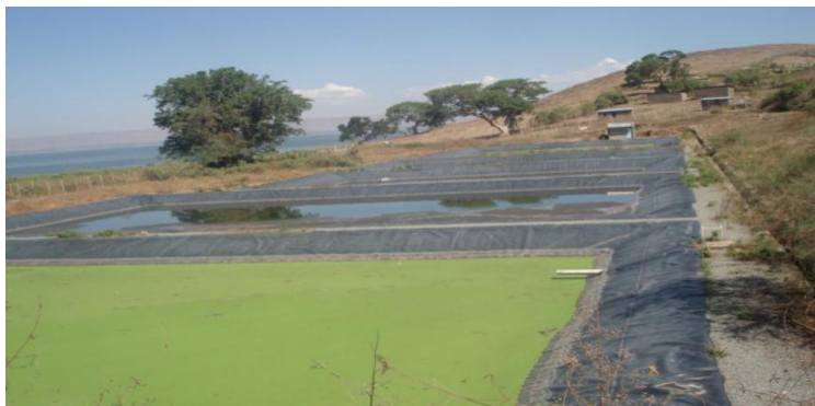
Figure 2.11 – WSPs at Hawassa Referral Hospital (Dires, 2008)
