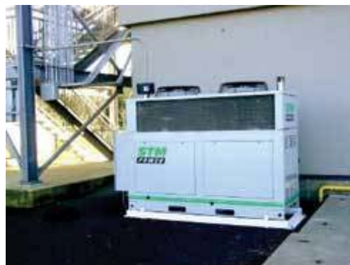
Figure 4-2. 55-kW Biogas-fueled Stirling engine cogeneration plant at the Corvallis wastewater treatment plant in Oregon.
