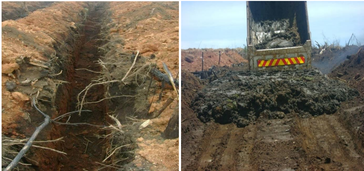
Figure 6.2 Prepared trench (left) and delivery of sludge from WWTW (right)
