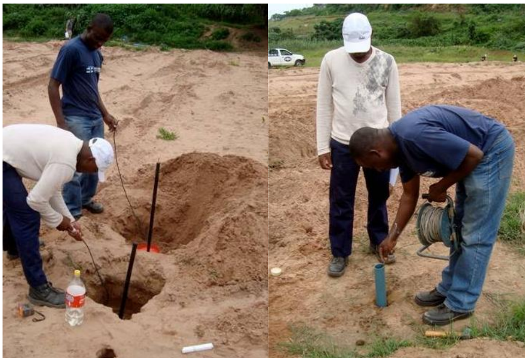
Figure 5.16 Installation of wetting front monitors (left) and monitoring of piezometers (right)
