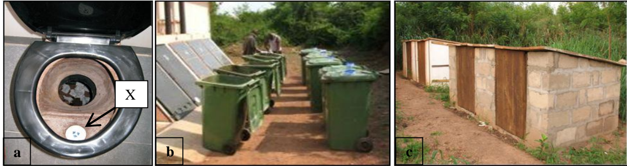
Figure 15: Dry toilet with fecal and urine separation (a) by means of membrane trap (X below), wheeled bins for transport of pre-fecal compost (b) and Chambers for composting(c)
