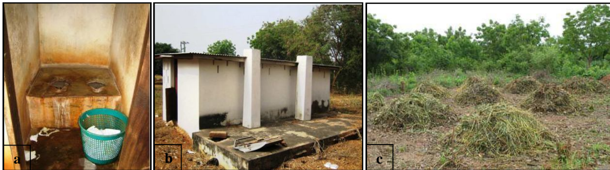
Figure 12: KVIP toilet chamber (with toilet pits) at J.J Nortey hall (a), back view of the KVIP (b), co-compost trials with sludge from KVIP(c).
