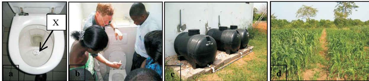
Figure 18: WSSFT with urine separation vents (X) (a), training of plumbers and cleaners (b), polyethylene urine storage tanks (c) and maize field on VVU campus applied with urine from the administration block (d).
