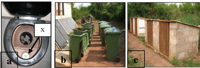
Fig 4: UDDT with faecal and urine separation (a) by means of membrane trap (X), wheeled bins for transport of pre-faecal compost (b) and Chambers for composting (c) (source: (a) Berger W., (b, c) Germer, J.).
