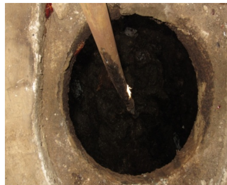
Non-homogeneity of pit latrine contents
