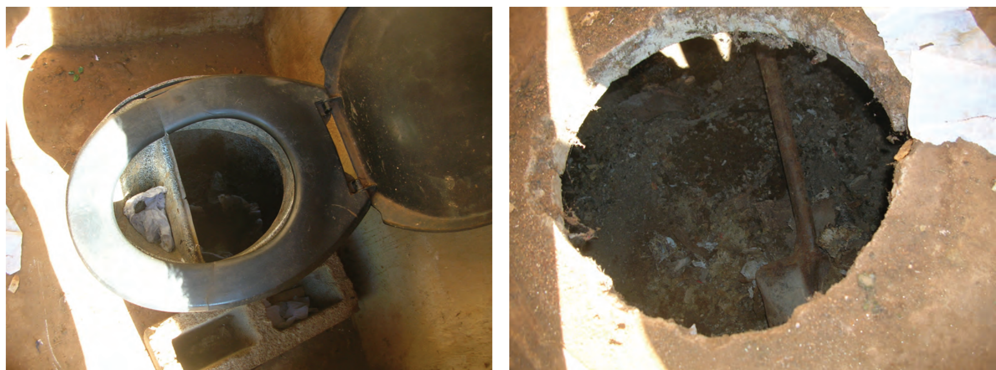
FIGURE 4 (a) Pedestal in position; (b) Pedestal removed—view into pit
