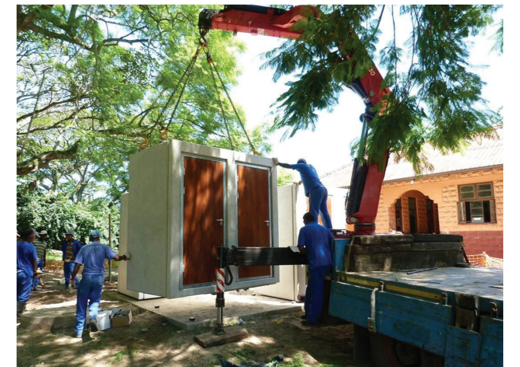
FIGURE 3 Installation of modules on-site
