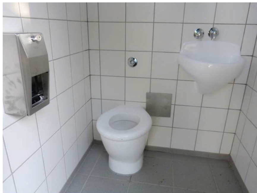
FIGURE 5 Inside a cubicle of an existing Hering toilet. Fixtures protrude through the back wall into the service corridor.
