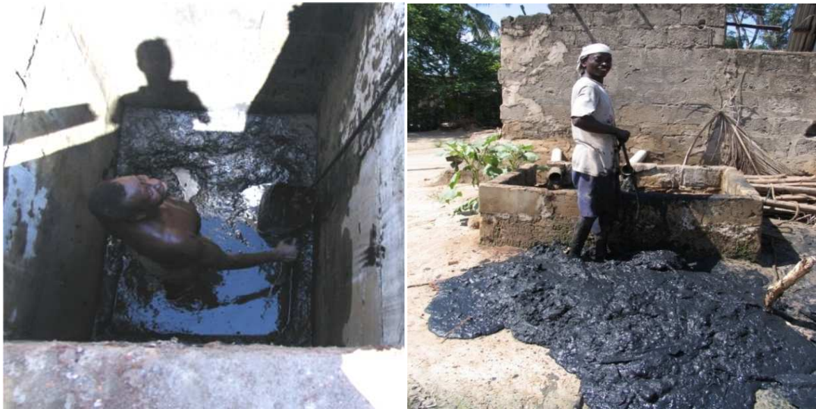
Figure 4.4 Manual pit emptying in Dar es Salaam (Sugden)
