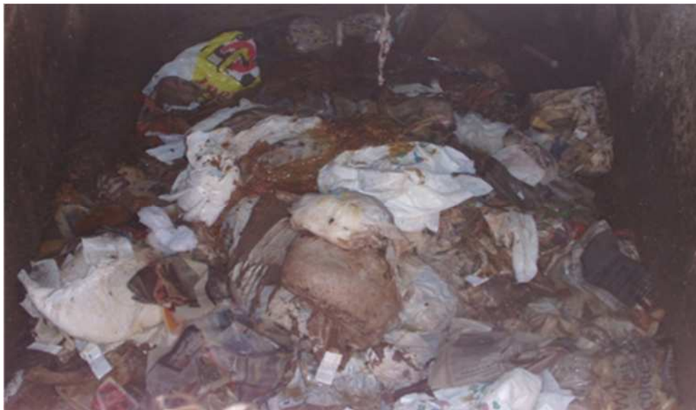
Figure 3.4 The use of the pit latrine for general household solid waste disposal shortens pit life and makes pit emptying by vacuum tanker almost impossible.
