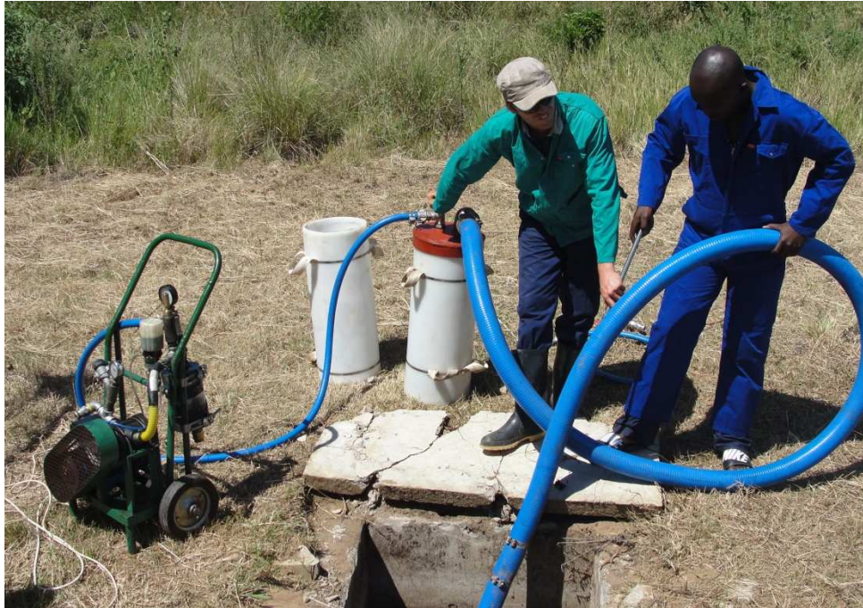
Figure 4.37 eVac emptying a pit using multiple pressure vessels with carrying handles
