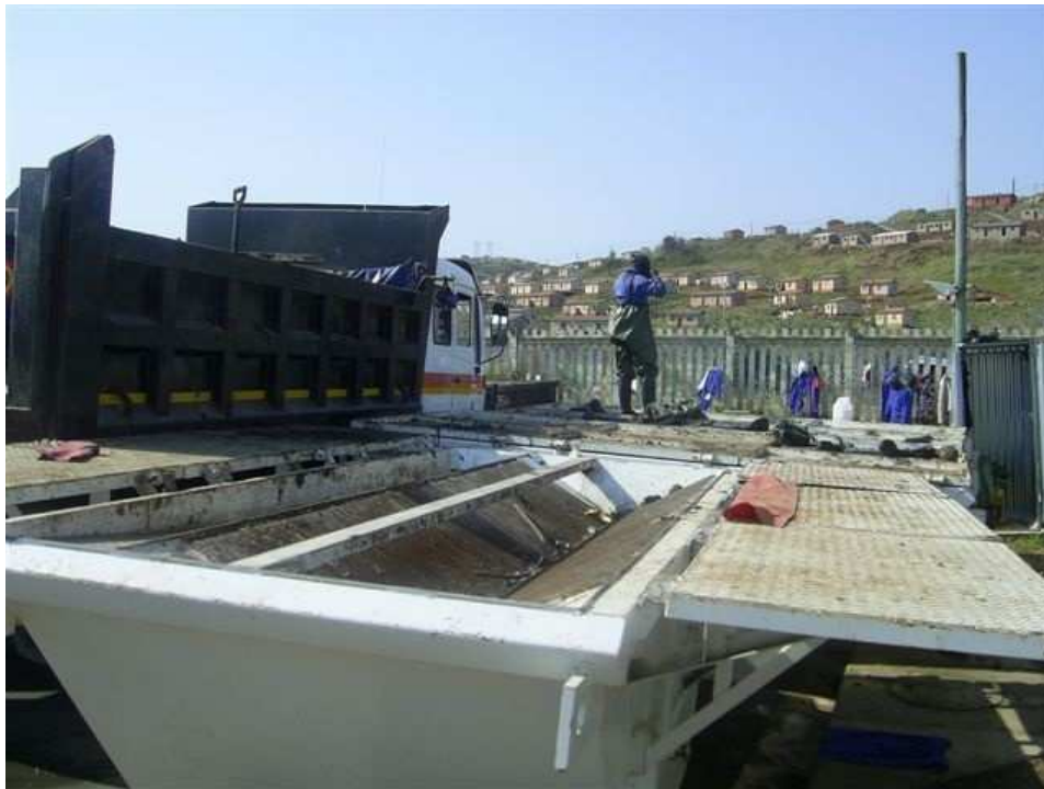
Figure 6.2 Screening trash out of sludge at WWTW (eThekweni Municipality) – it was found that the addition of pit latrine sludge at WWTWs quickly overloaded the works and this practice was discontinued
