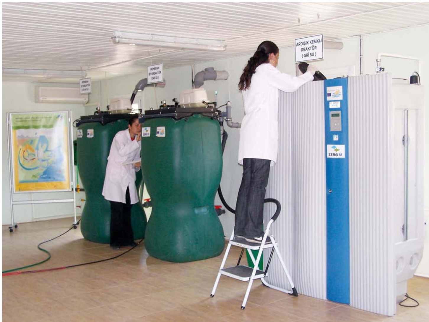
▲ Figure 7: MEMBRANE BIOREACTOR
