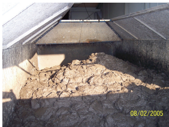
FIGURE 9-1 DEWATERED SLUDGE READY FOR TRANSPORT
