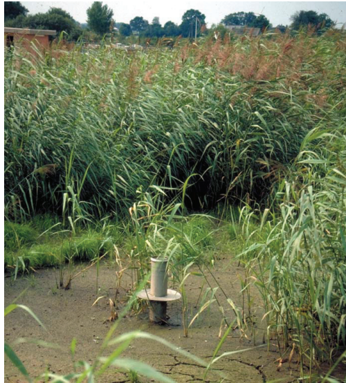
FIGURE 4-19 SLUDGE MINERALIZATION BEDS WITH VERTICAL FLOW
