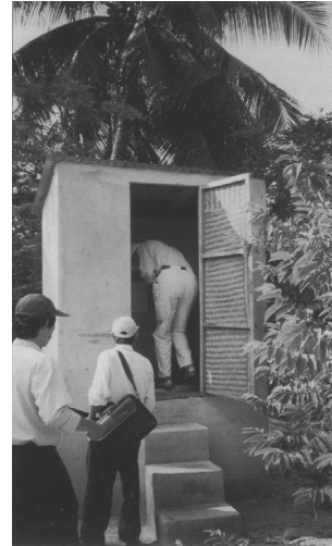
Elevated Urine – Separating toilet in VN
