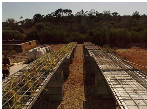
FIGURE 5-4 EPUVALISATION CHANNELS
