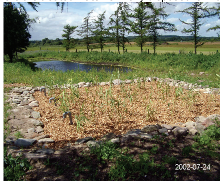
FIGURE 4-24 INSULATED PLANTED BED AFTER FIRST MONTH OF OPERATION The lake where the treated water is finally disposed is in the background
