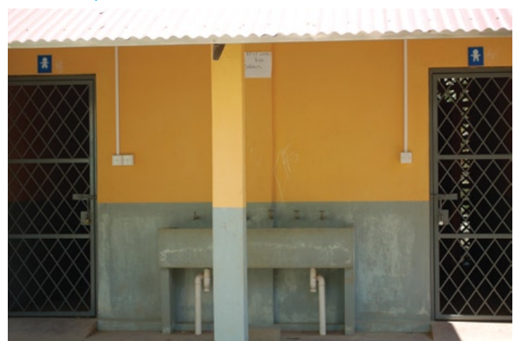
FIGURE 5.4 WASH facility locked due to lack of water, Timor-Leste
