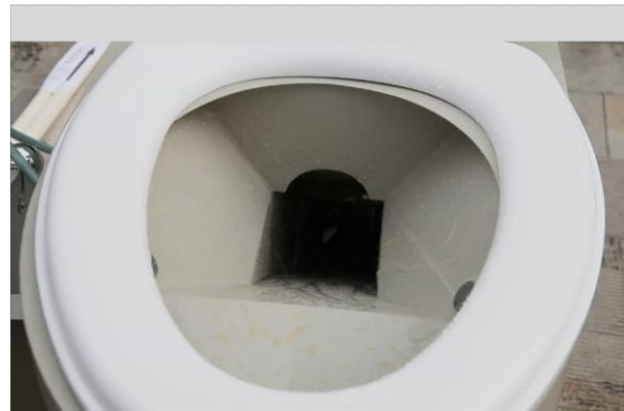
Distilled water from the liquid part of the fecal sludge used to clean the toilet bowl using a pressurizing pump.
