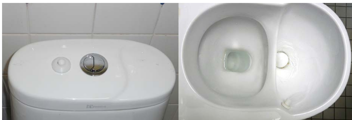
Figure 10: (a) The Dubbletten flushing mechanism - the white button for rinsing the urine bowl, and silver half and full flush buttons activate the flushing of the rear bowl (b) Water jet rinsing the urine bowl
