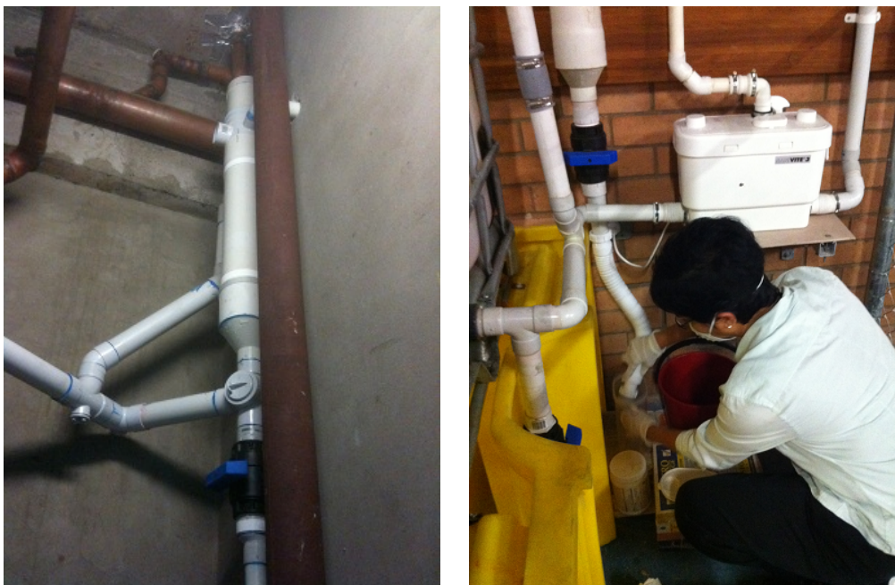
Figure 41: Urine sampling set up for UDT (left), and sample collection from the waterless urinals (right)
