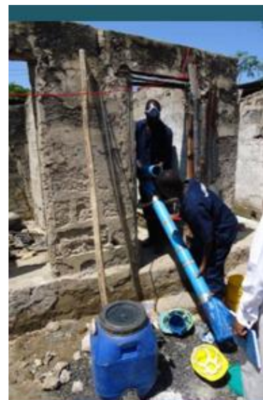
Fig 3: A hygienic emptying team in action in Dar es Salaam © Schaub-Jones
