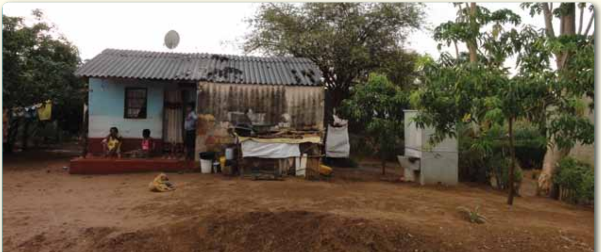
Typical household with new toilet (right) at Libuyu project, Livingstone
