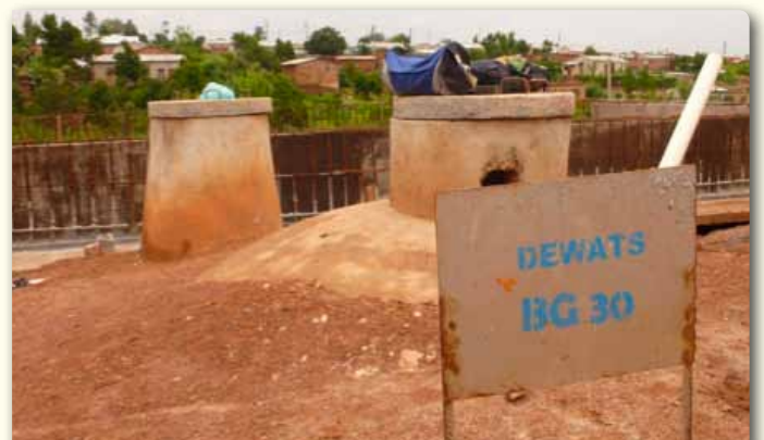
Construction of decentralised waste water treatment system at Kandundu project in Solwezi
