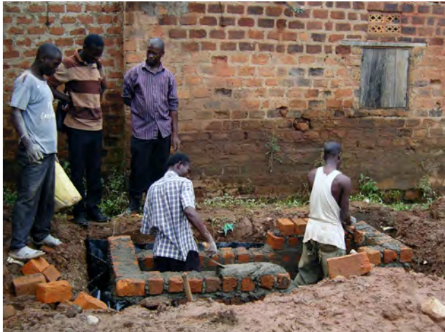
Fig 1 Construction of raised double-stance VIP latrines in Bwaise Division, Kampala in 2012. © Roman Grüter
