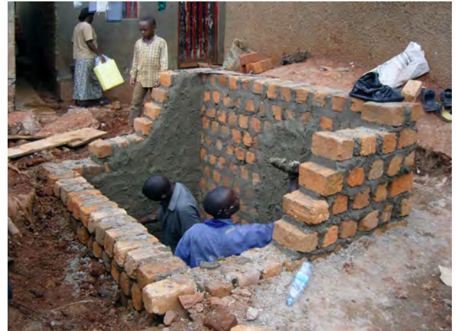
Fig 1 Construction of raised double-stance VIP latrines in Bwaise Division, Kampala in 2012. © Roman Grüter
