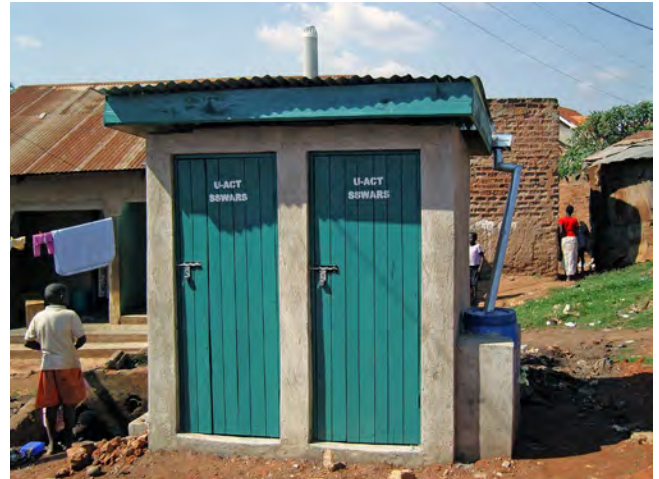
Fig. 3 Ground-level VIP latrine
