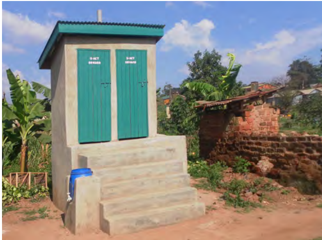
Fig. 2 Raised VIP latrine
