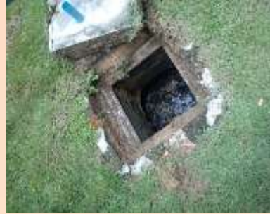
(a) Opened septic tank cover
