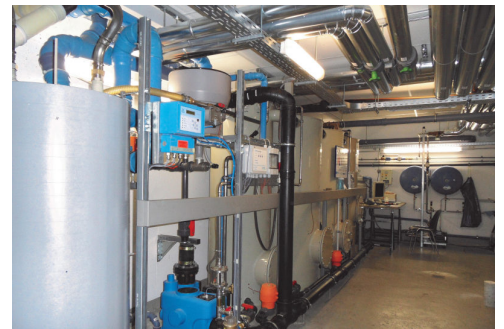
Photo 2: Greywater recycling combined with heat recovery. The combined system is placed in the basement where the building's heating system is also found, occupying an area of 9 m 2 (approx. 0.1 m 2 /person).
