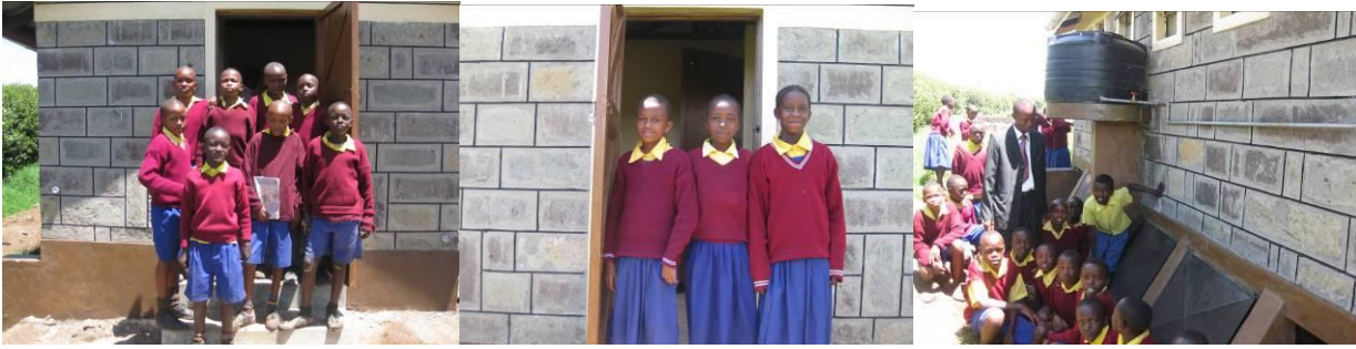
Figure 2: Pictures showing the quality of materials and work done
