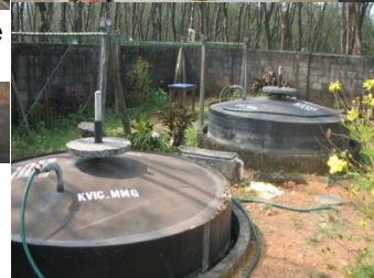
Gas Pipe line
