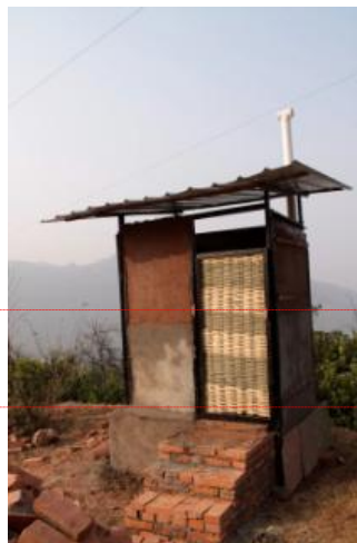
Fig. 4: Image example (Nov. 2008 during the construction)
