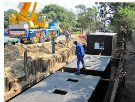
Multi-chambered ABR under construction
