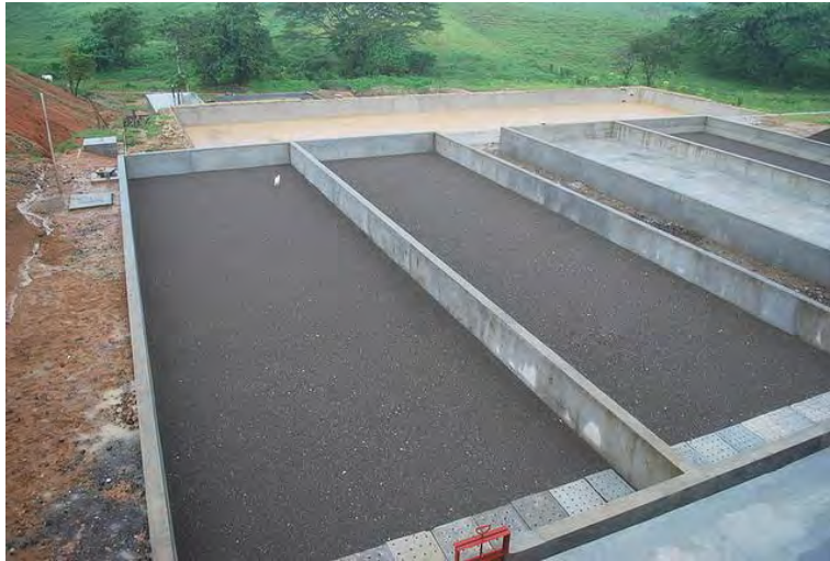
Drying beds located at the Bayawan City Waste Management and Ecology Center
