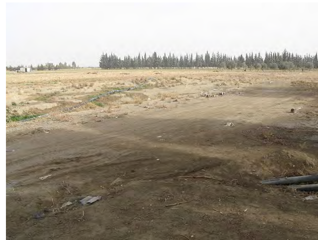
Pipe with treated effluent to irrigation site
