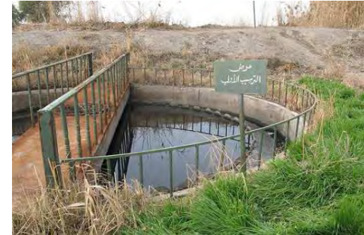
Circular primary settling tank
