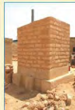
3. Double vault with sub- and superstructure in adobe (US$ 279)
