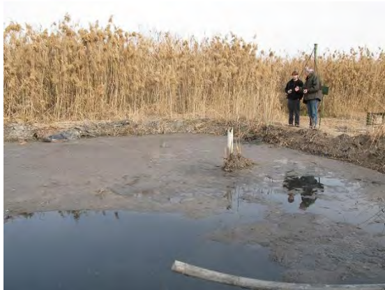
Primary sludge drying bed in front of reed bed. At the front you can see the sludge pipe from the primary settling tank.
