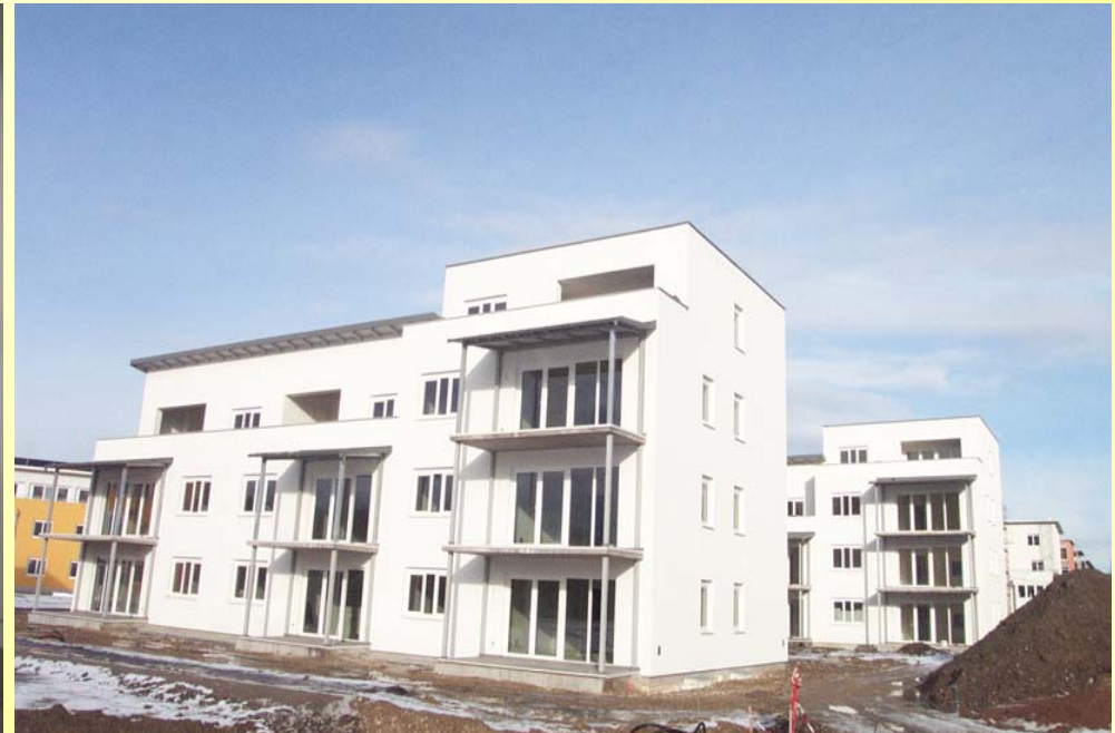
Buildings (photo: Otterwasser GmbH)
