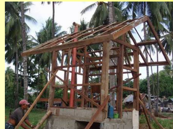
Construction and inauguration of the UDD-Toilet
