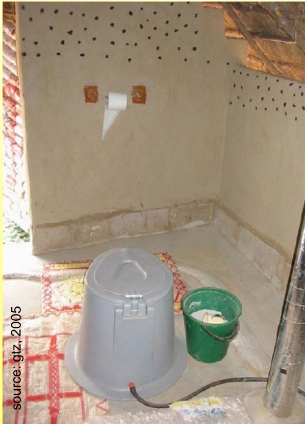
urine diversion toilet made out of plastic
